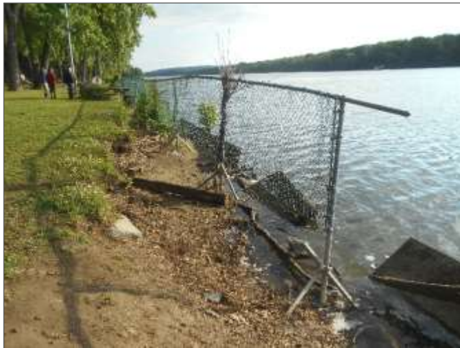
Photograph 7: View looking south at the timber cribbing with riprap and concrete capping.
