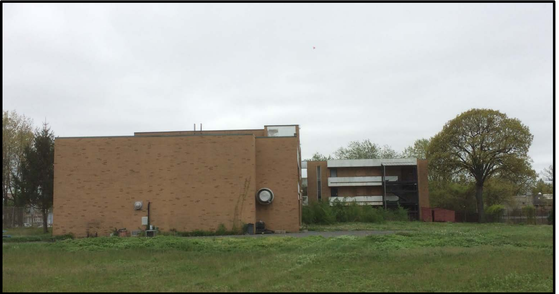
Building 165 (on left) and 166 (on right) north facade (facing south; April 2016).
