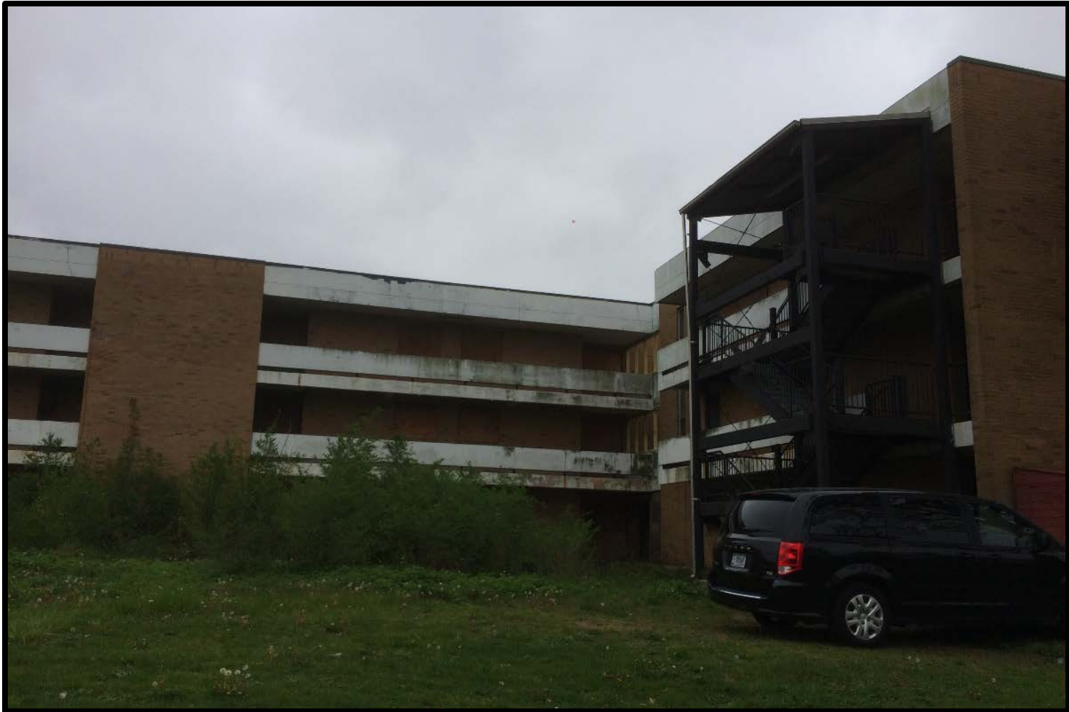
Building 165 (on left) and 166 (on right), west facade (facing east April 2016).
