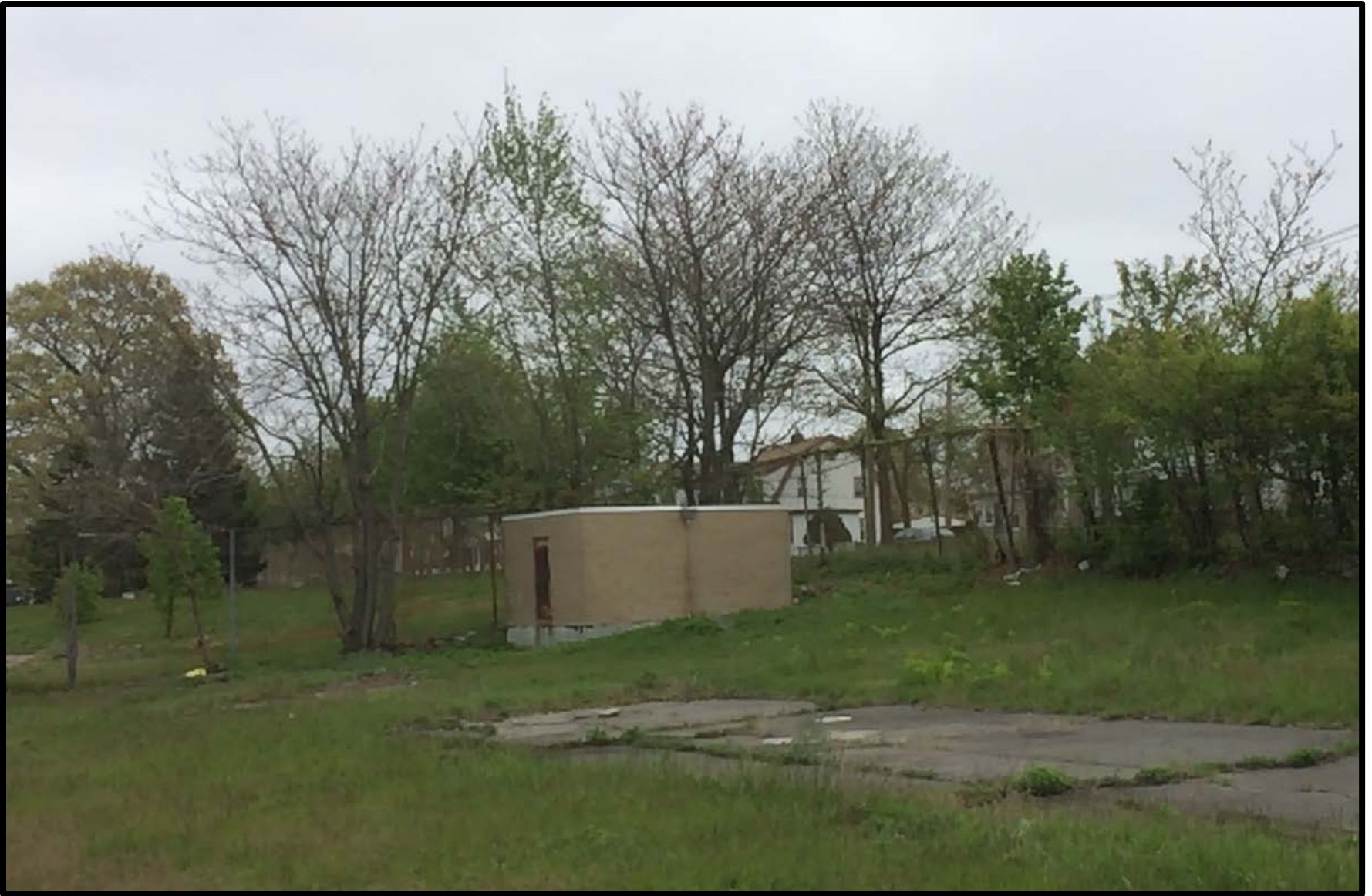
Utility Building on the northeast portion of the property (facing northeast, April 2016).
