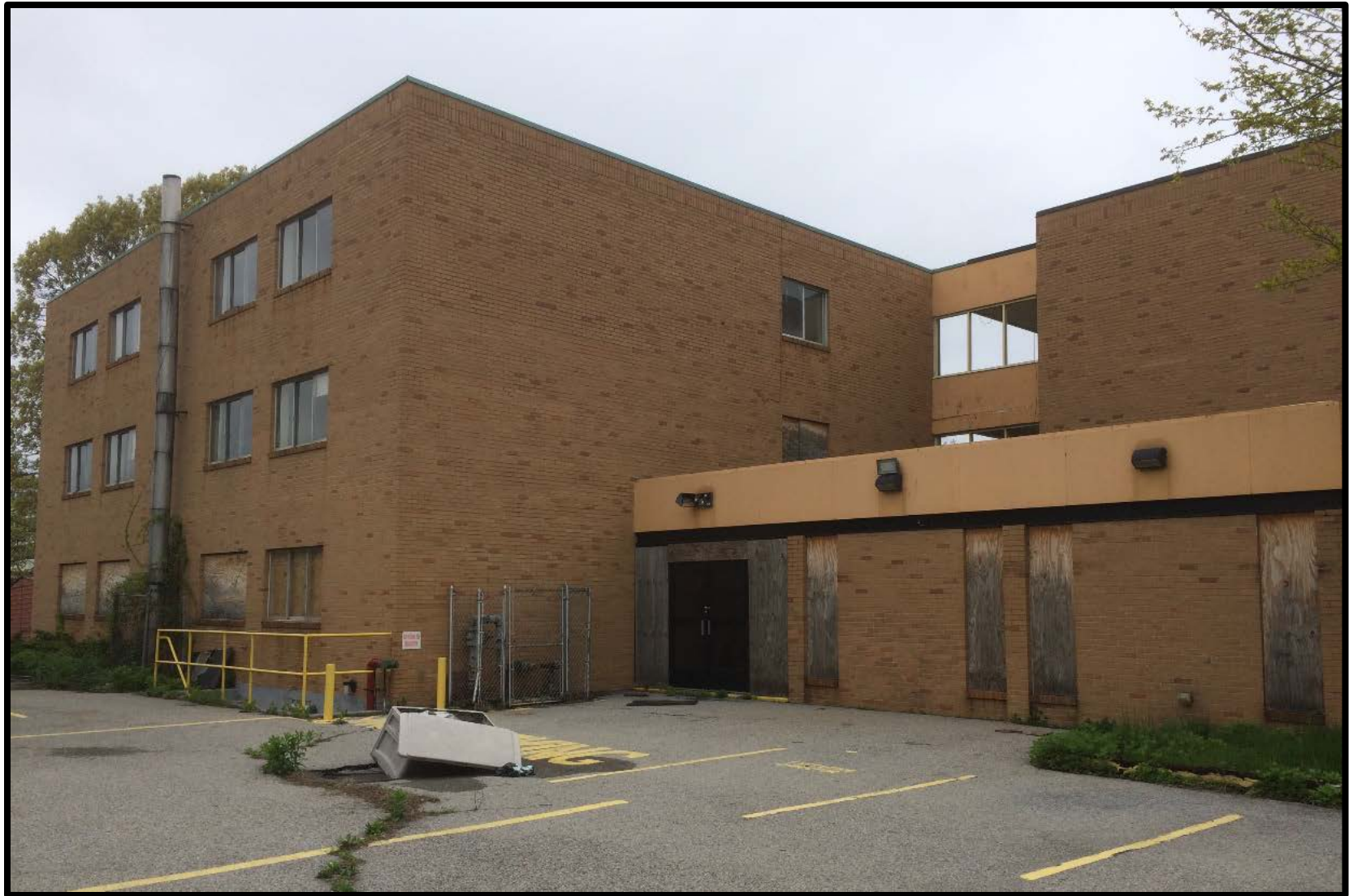
Buildings 165 (right) and 166 (left), south facade (facing north; April 2016).
