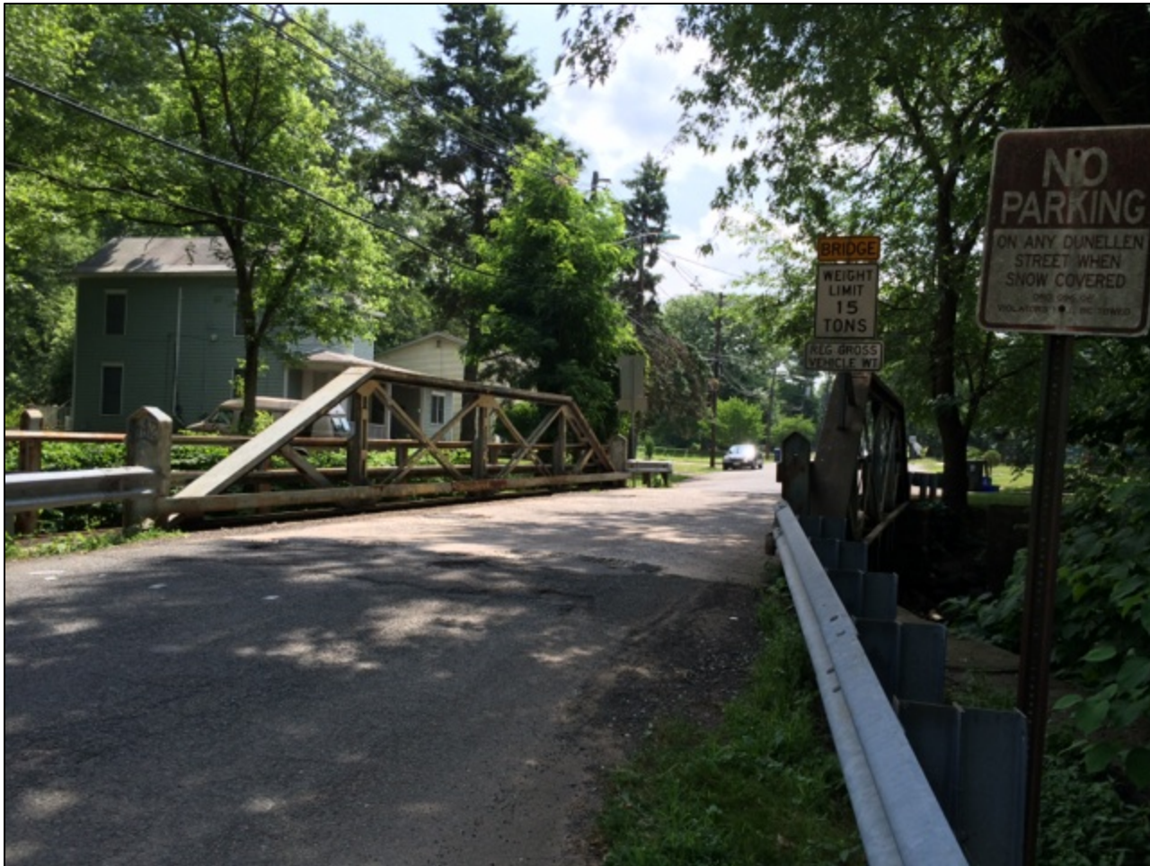
Enclosure 4. Jefferson Avenue Bridge view looking southeast. Photographer: Lynn Rakos, July 2014.
