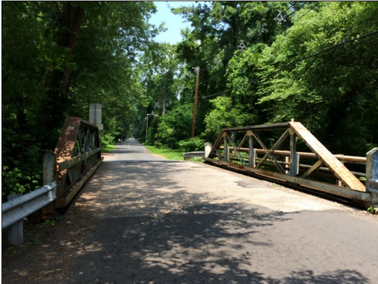
Enclosure 5. Jefferson Avenue Bridge view looking northeast. Photographer: Lynn Rakos, July 2014.
