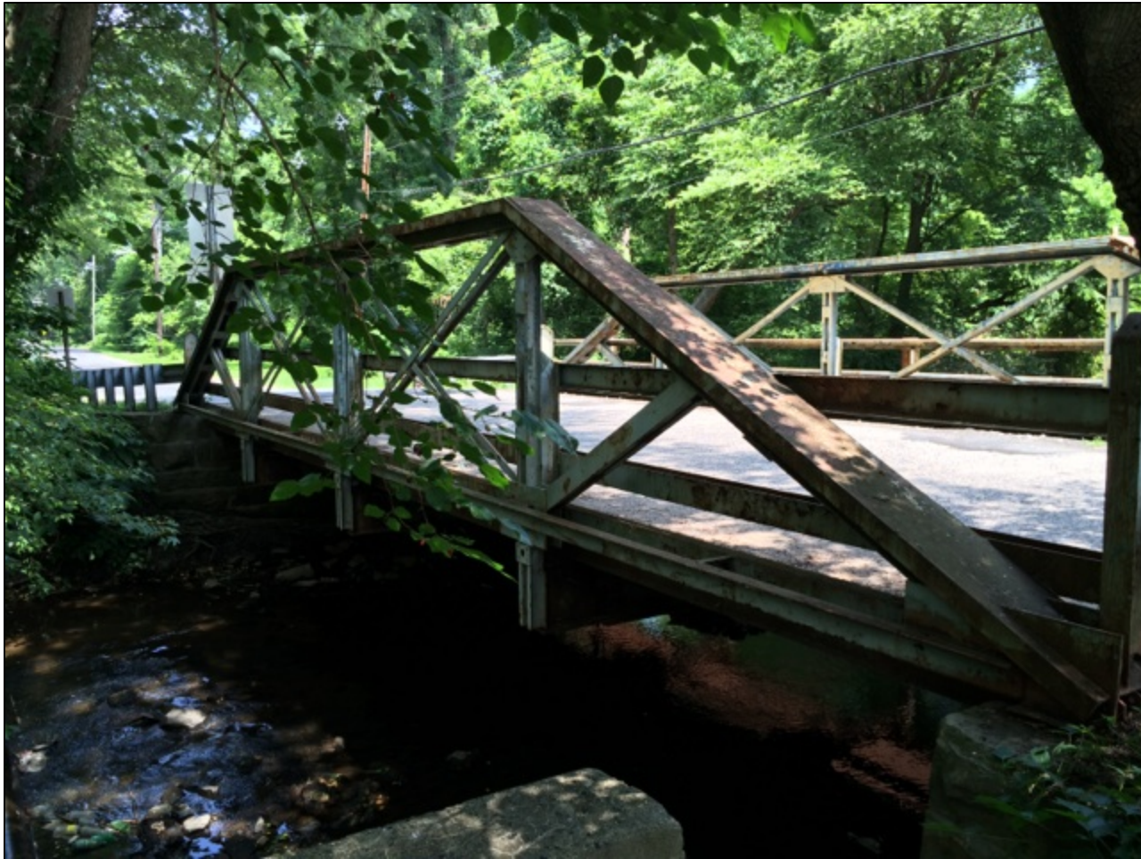
Enclosure 6. Jefferson Avenue Bridge view looking north. Photographer: Lynn Rakos, July 2014.
