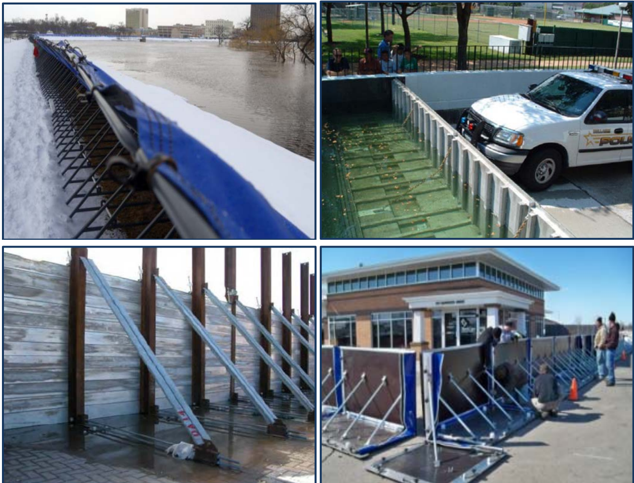
Figure 25: Deployable ringwall concepts. Counter clockwise from top left: Portadam, FloodBreak, AquaFence, and a rapid deployment floodwall.
