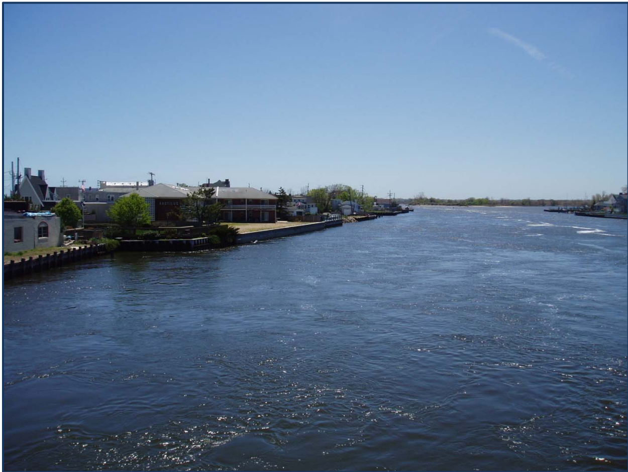
Figure 22: Typical bulkhead along the Shrewsbury River in Sea Bright, 2014. A floodwall would be visually similar to it, but would be higher in elevation.
