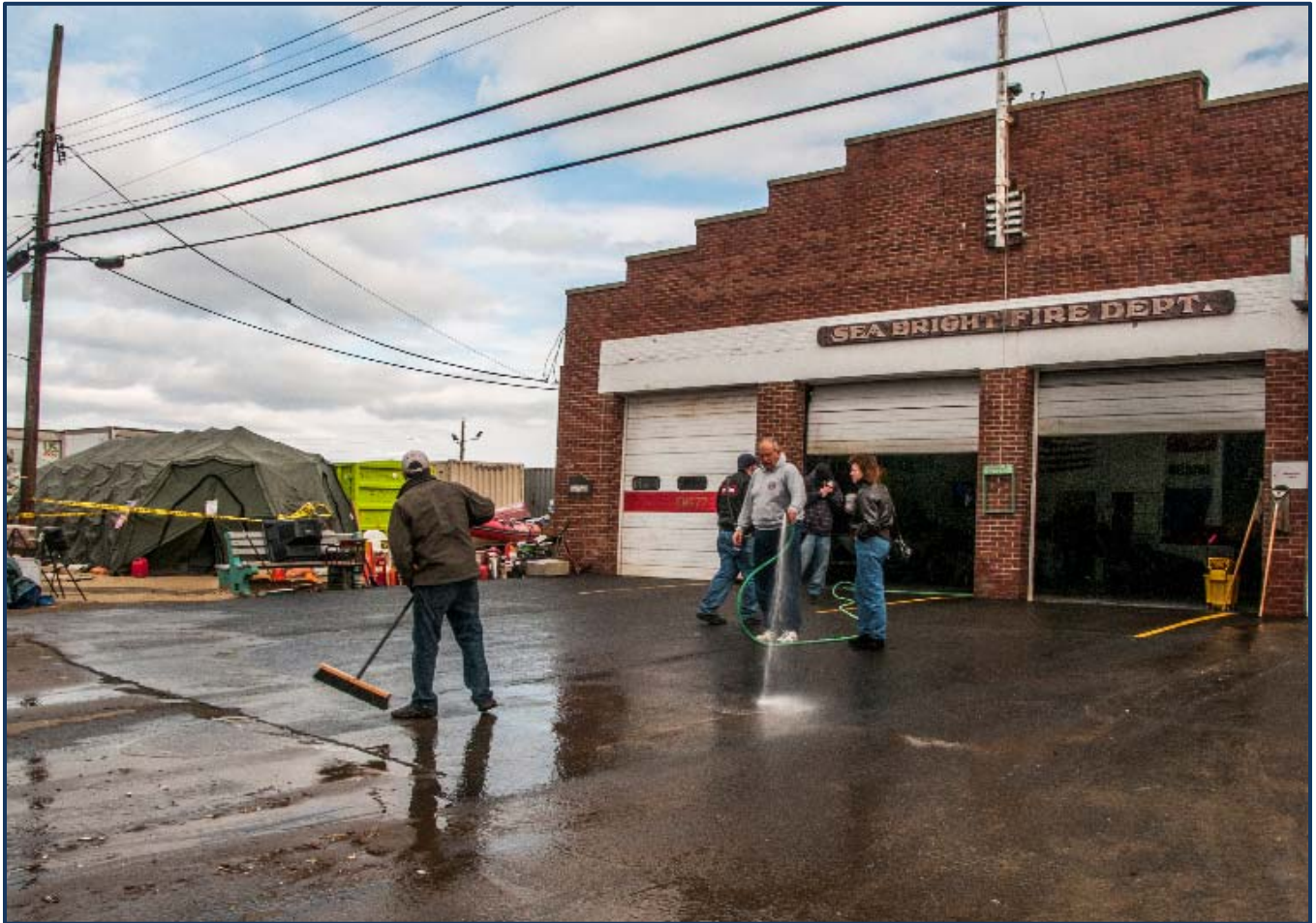
Figure 10: Firefighters clean the Sea Bright fire station after Hurricane Sandy, 2012.
