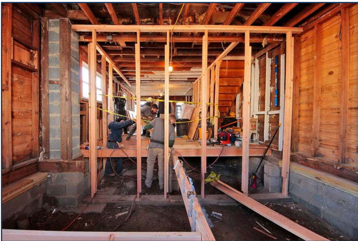
Figure 29: Rebuilding flooded home on New Street, 2014.
