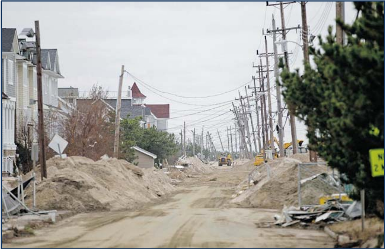
Sea Bright, New Jersey after Hurricane Sandy, November 2012.
