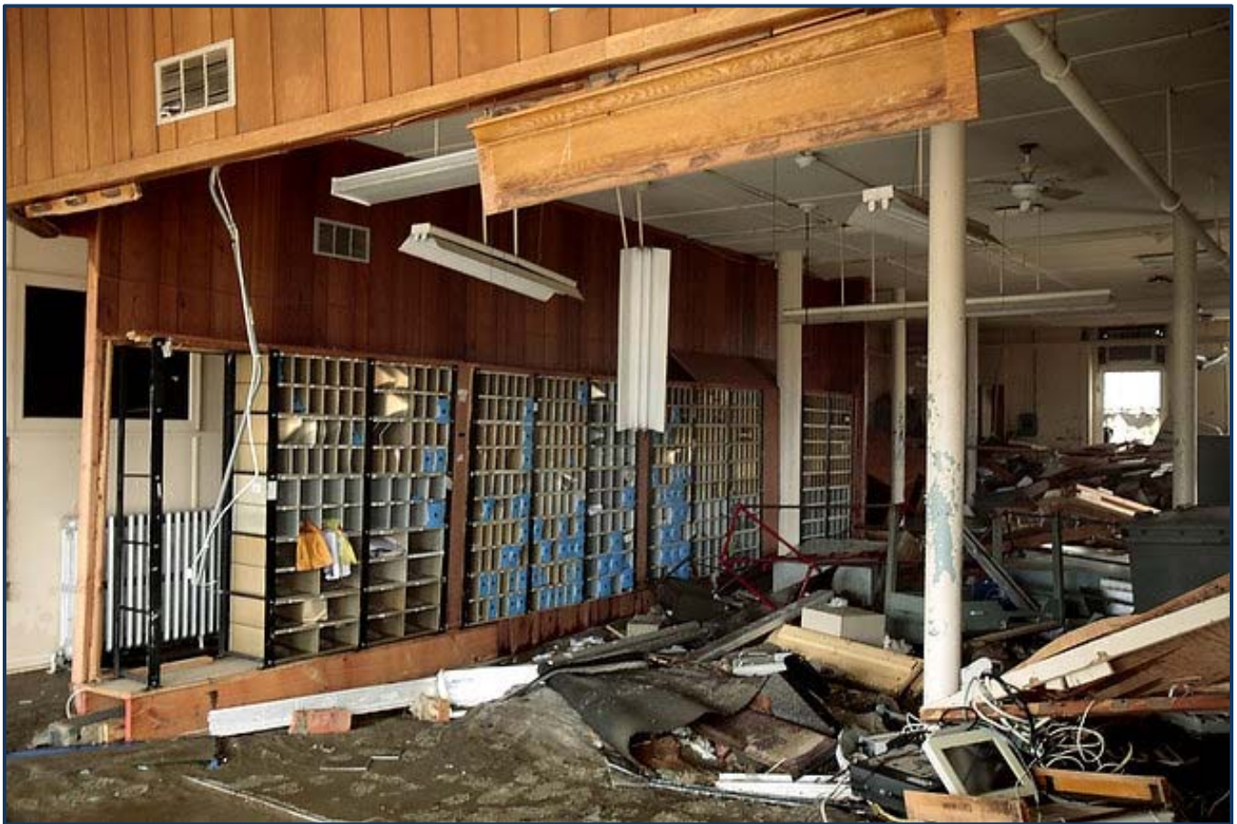
Figure 21: Sea Bright post office after Hurricane Sandy, 2012.
