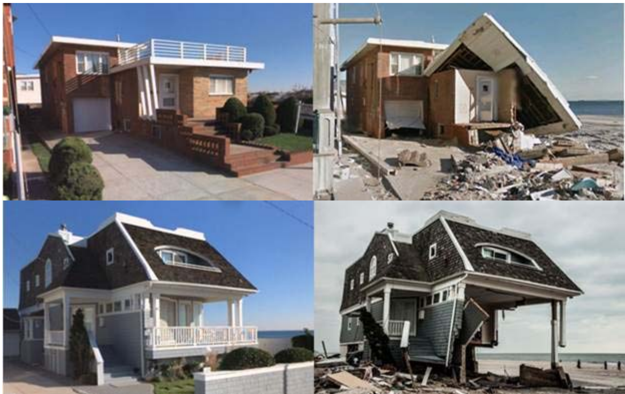
Figure 5: Before and After Photos of Rockaway Beach Structures Damaged by Hurricane Sandy
