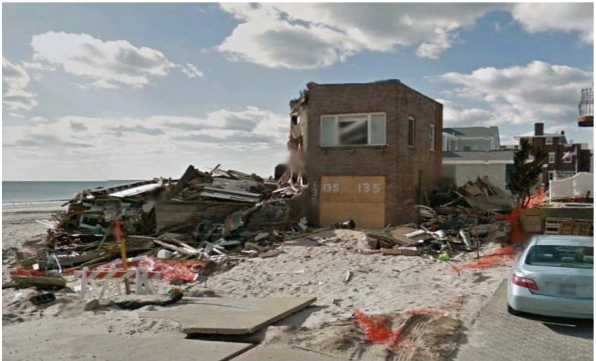
Figure 4: Rockaway Beach Structure Damaged by Hurricane Sandy
