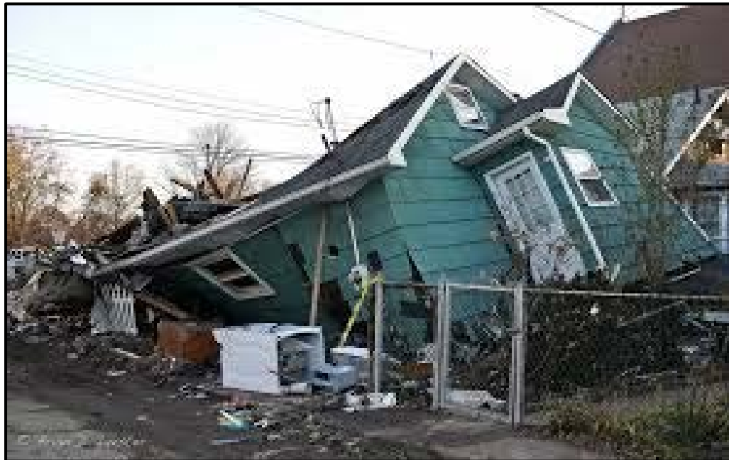
Figure 13 – Typical Hurricane Sandy Damage
