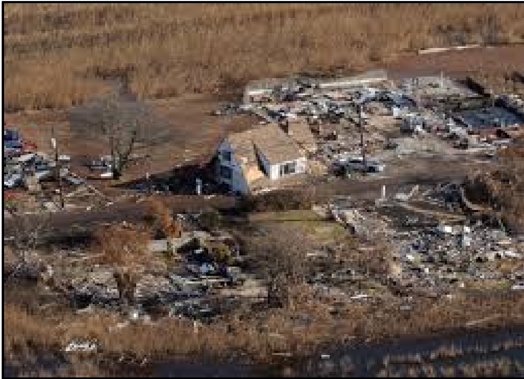
Figure 12 – Typical Hurricane Sandy Damage
