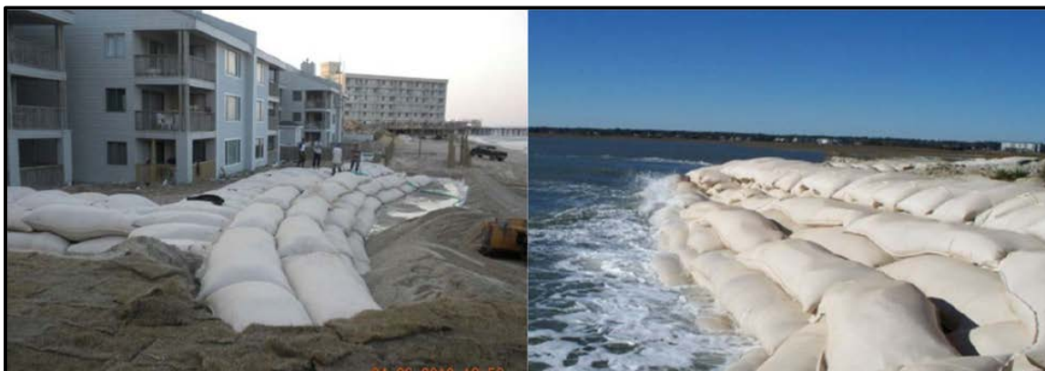
Figure 5: Geobag Example Installations
