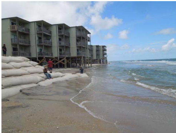
Revetment Approaching Last 2 Buildings
