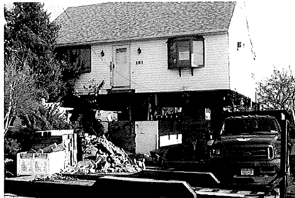
Above: Residential structure elevation project underway in the Village of Freeport
