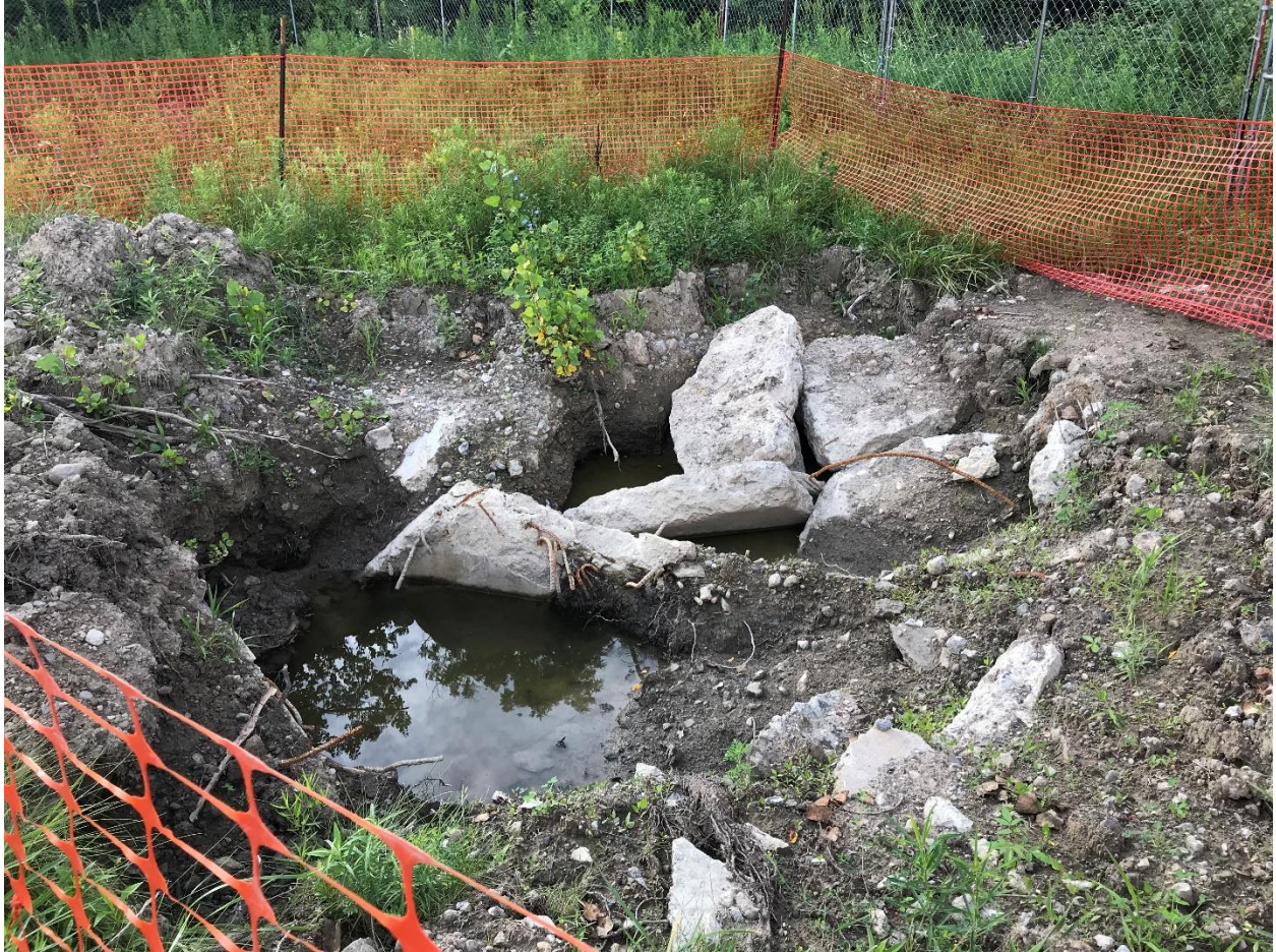
Figure #2 – Silo 6 Stair Entry Filled with Concrete Debris and Water
