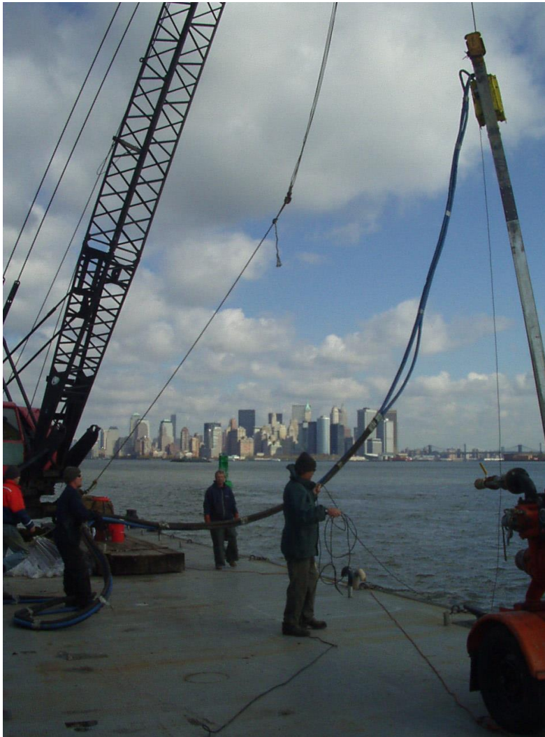
Figure 5.11: Coring along Liberty Island.
