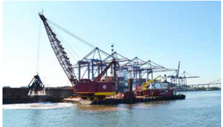
To allow large ships to safely transit the shipping channel, a dredge deepens the Arthur Kill Channel approaching the New York Container Terminal in the waters off of Elizabeth, N.J. and Staten Island, N.Y. (photo by Vince Elias, New York District)
