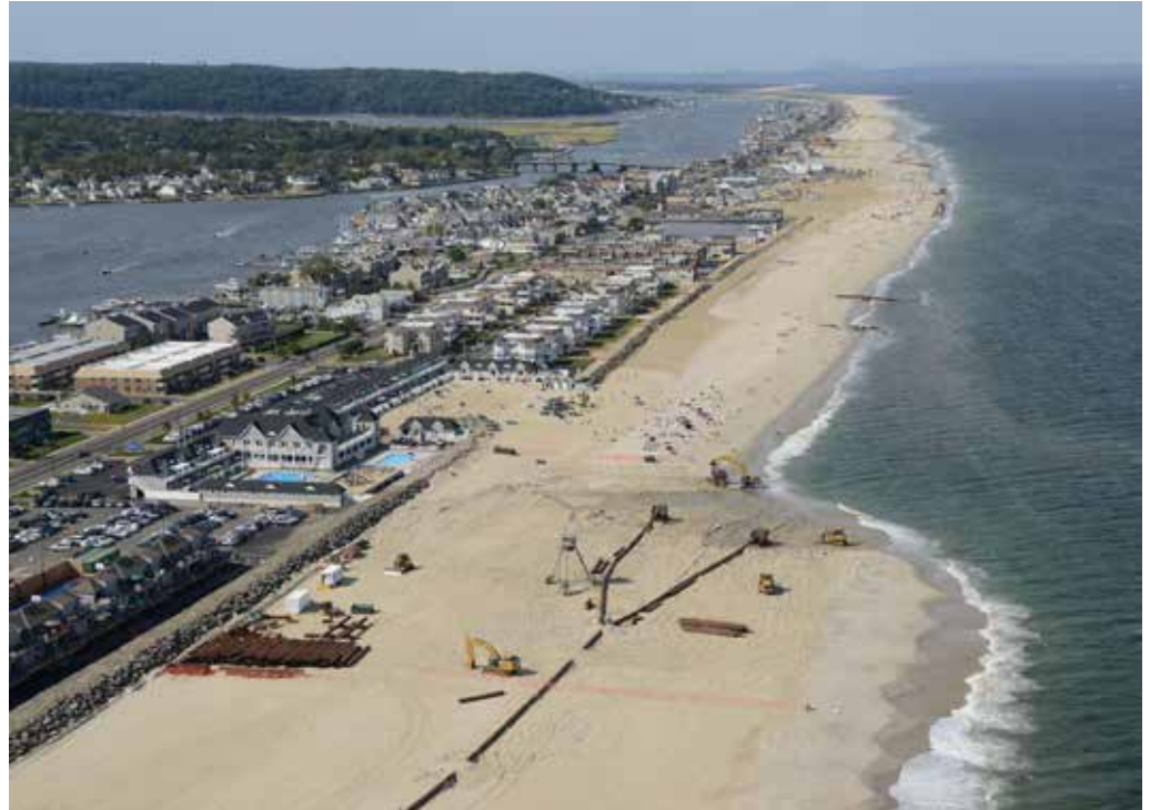
Sea Bright, N.J., on September 7, 2013 during post-Sandy repair and restore work, was one of several coastal communities where the Corps of Engineers managed work to increase the height and width of previously constructed beach berms in 2013 impacted by Hurricane Sandy at the end of 2012. (File Photo)
