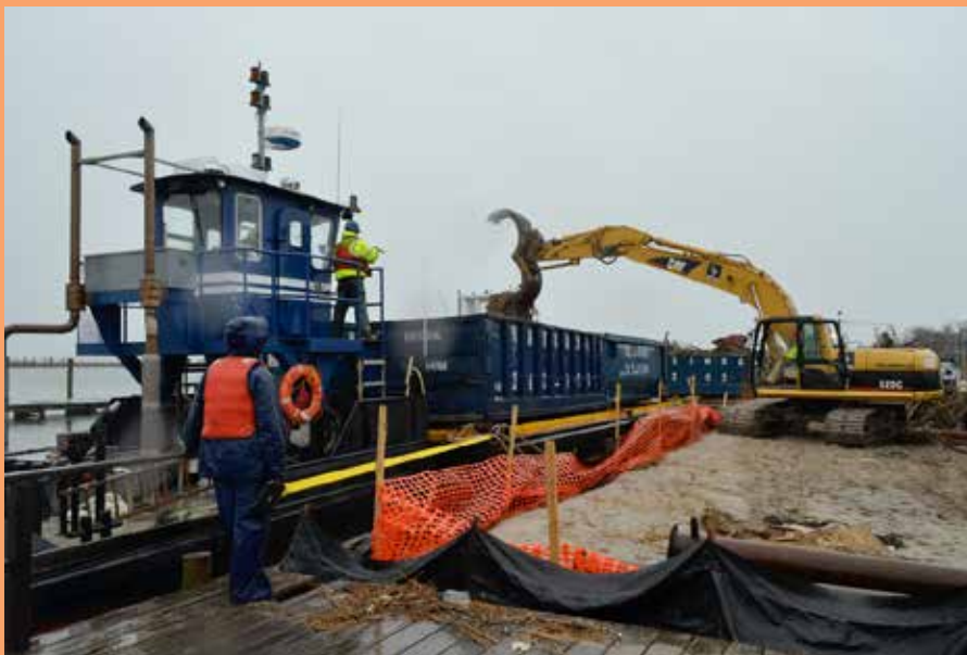
Due to the remote nature of Fire Island and the limited vehicular access, debris was loaded onto barges for disposal during post-Sandy debris removal efforts there in early 2013. (photo by Chris Gray-Garcia, New York RFO)
