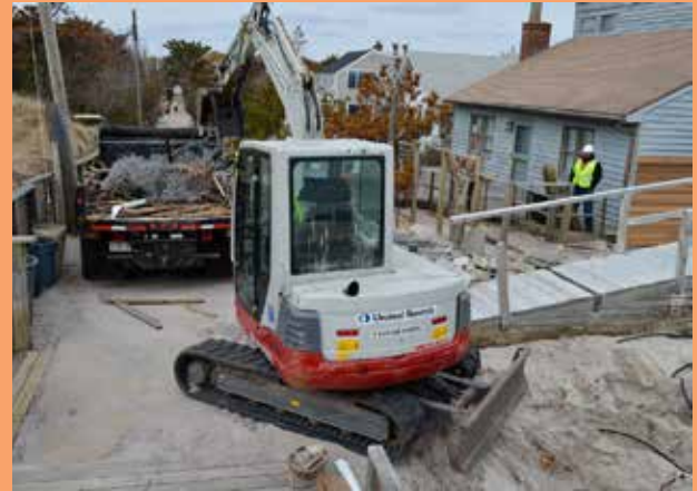
Crews worked and moved in limited spaces around homes on Fire Island during post-Sandy debris removal efforts there in early 2013. (photo by Chris Gray Garcia, New York RFO)
