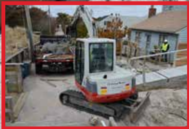
Finishing Debris Removal Mission in 2013, pg 4
