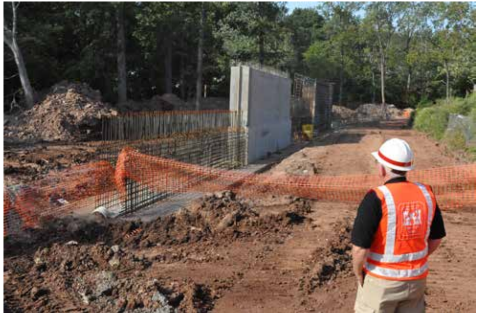
Timothy Yarger, of New York District's Construction Division, looks at early progress in late 2012 on the construction of a floodwall in Middlesex County, N.J., that is part of the larger, multi-county Green Brook Flood Risk Reduction Project the Corps is building in partnership with the state of New Jersey. While major construction for the nearby Bound Brook portion of the project in Somerset County was completed in late 2012, work in nearby Middlesex County on elements like this one ramped up and hit full stride throughout 2013. (photo by Chris Gardner, New York District)
