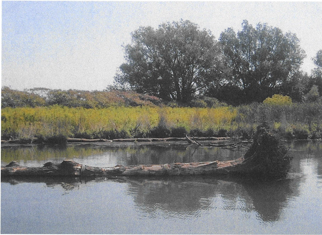
Figure A2. Log Breakwall in Niagara River. Photo by Tim DePriest, NYSDEC.
