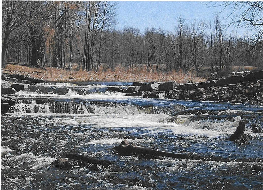
Figure 6. Step pool structures installed after dam removal allow fish passage but retain sediment in old impoundment.
