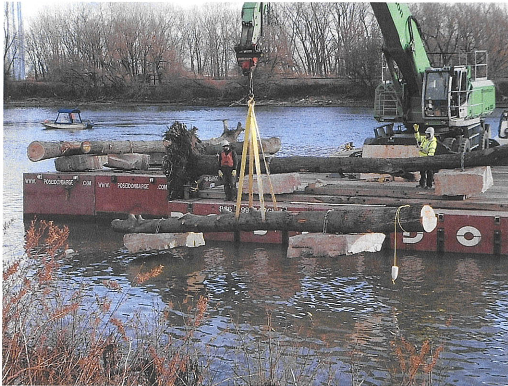
Figure 4. Log Breakwall Installation. Photo by Tim DePriest, NYSDEC.
