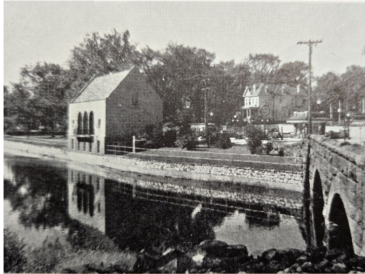
Both the picturesque building constructed in the 1920s to house a sewage ejector station and stone retaining walls along the New York Side of the Byram River complimented the Byram Bridge at right edge of photograph (1933).
