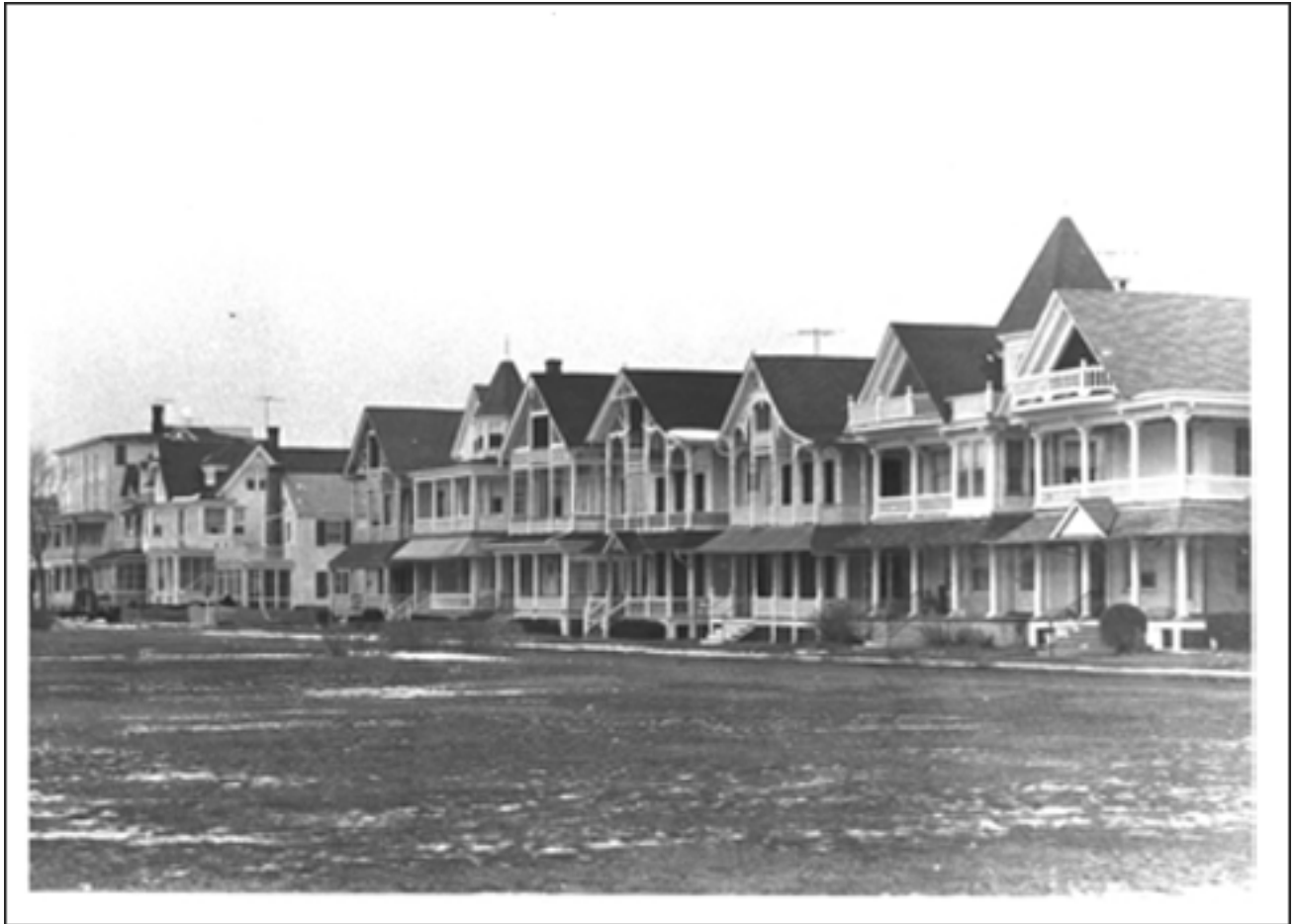
Figure 9: View of Ocean Grove Camp Meeting Association Historic District (NRHP Nomination Form 76001170)
