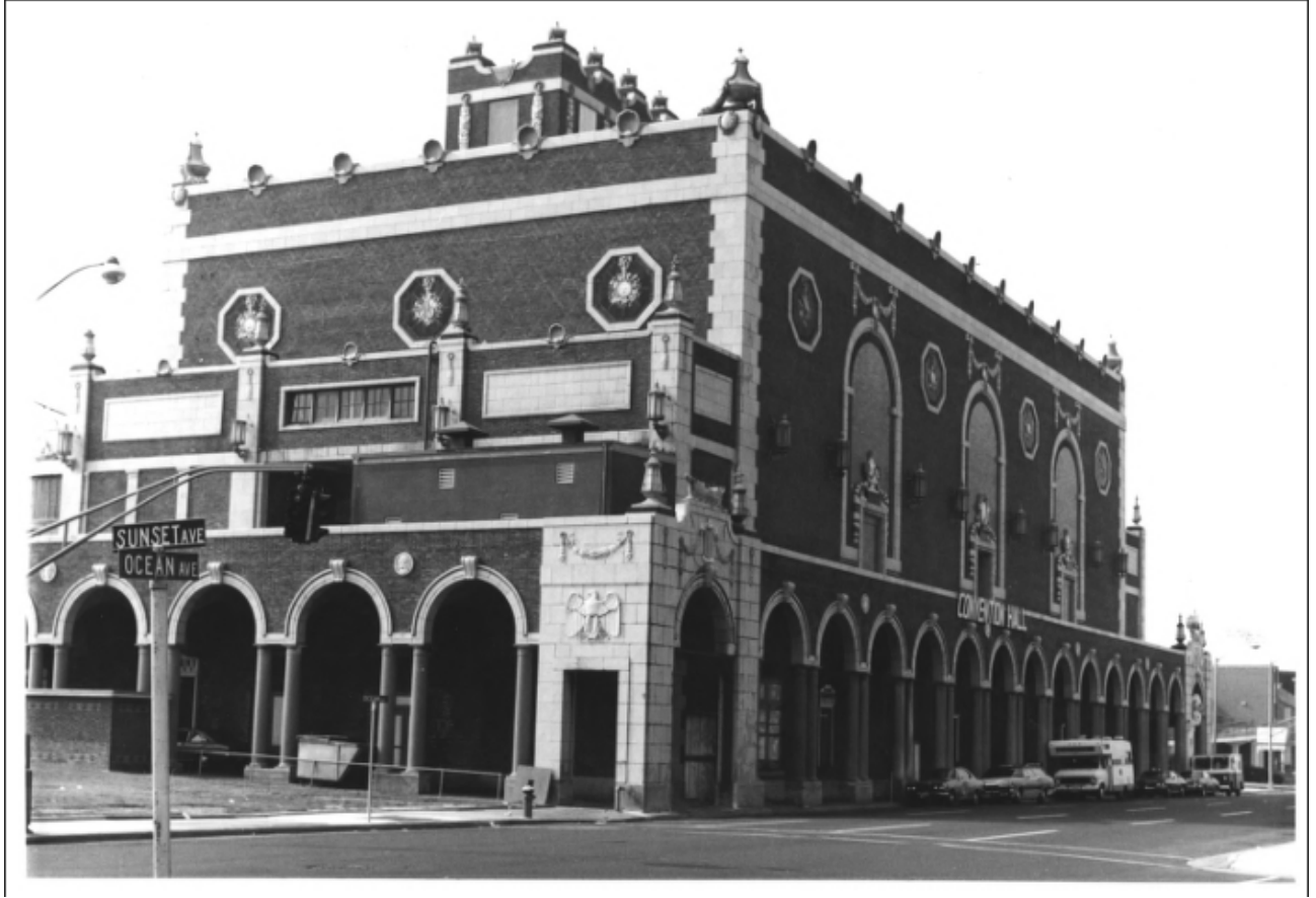
Figure 11: Photo of The Asbury Park Convention Hall (NJDEP Historic Site Inventory Form No. 1303-33)
