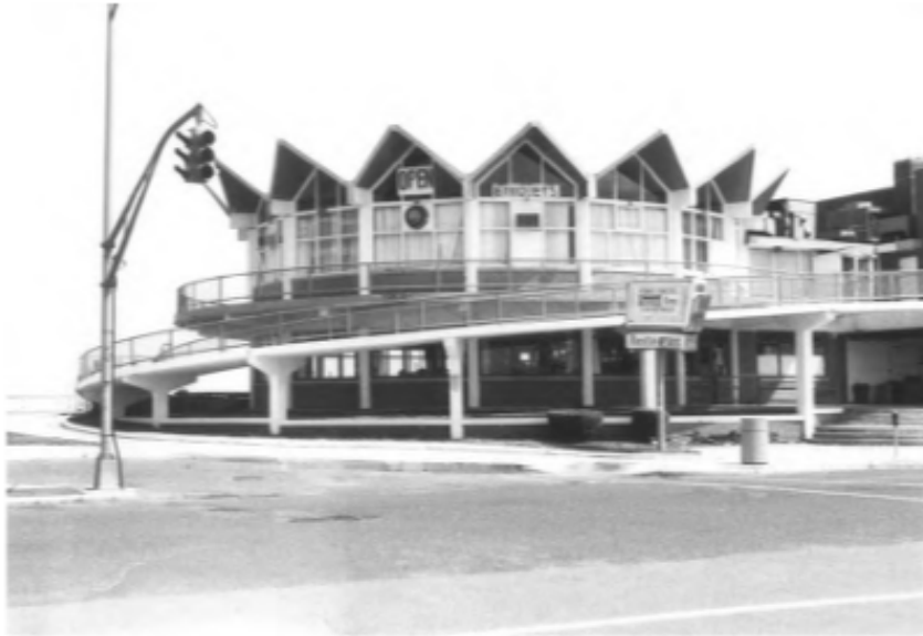
Howard Johnson Pavilion, view east from Ocean Ave. Photograph 2000
