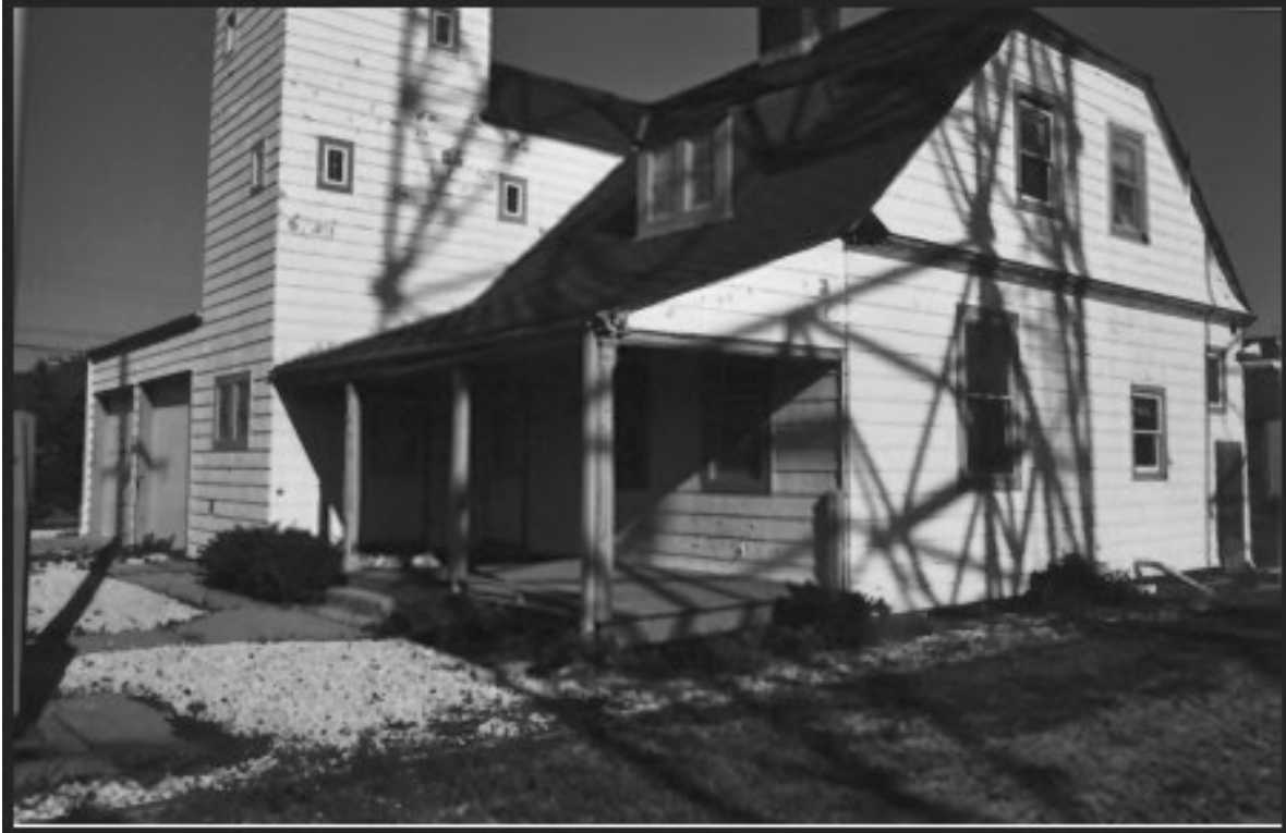
Figure 16: Photo of the side of Life Saving Station #9 (NRHP Registration Form 07-0103-3SA135)
