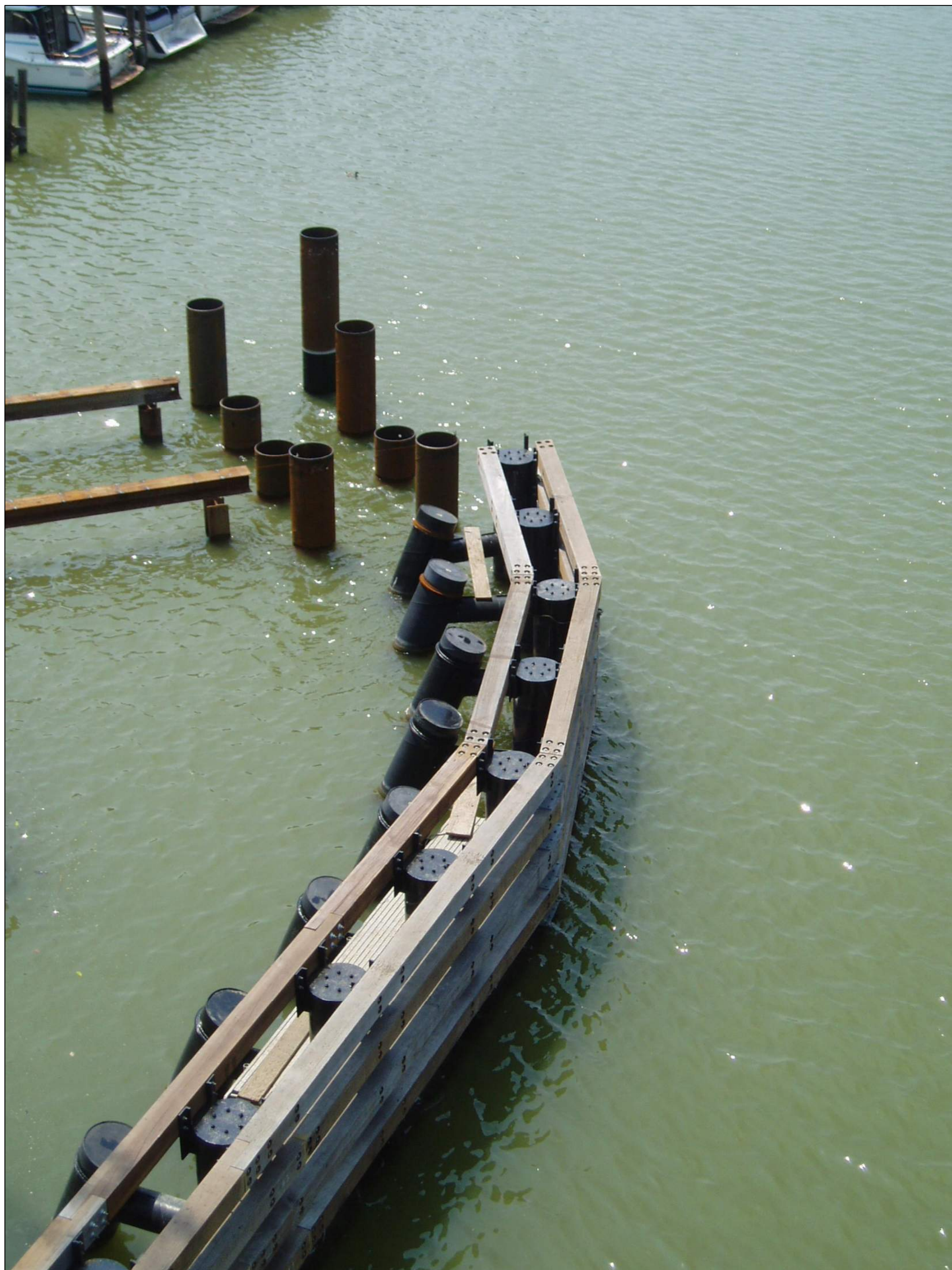
PHOTO REFERENCE - GUIDE FENDER SYSTEM
