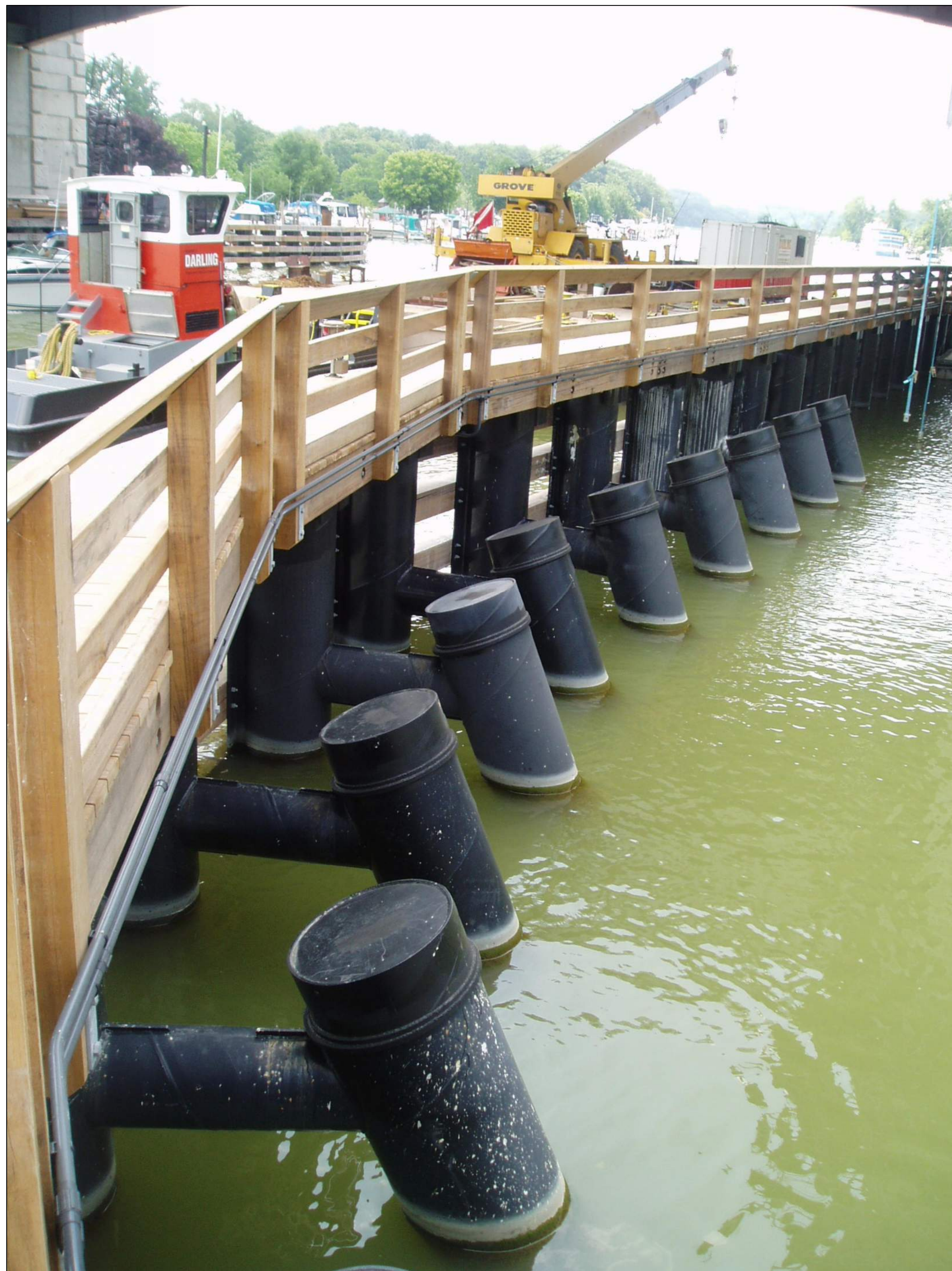
D3 R-004 PHOTO REFERENCE - GUIDE FENDER SYSTEM
