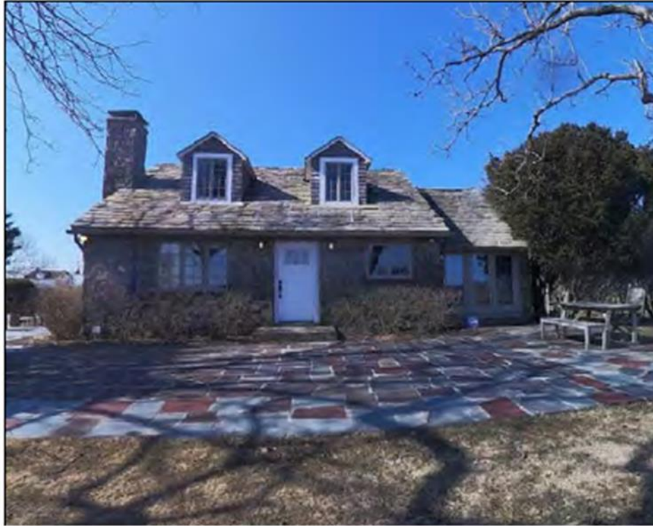
Figure 7: 502 Riviera Drive, Mastic beach (Dewberry 2025)
