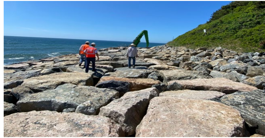
Construction of new revetment (Jun 2022)
