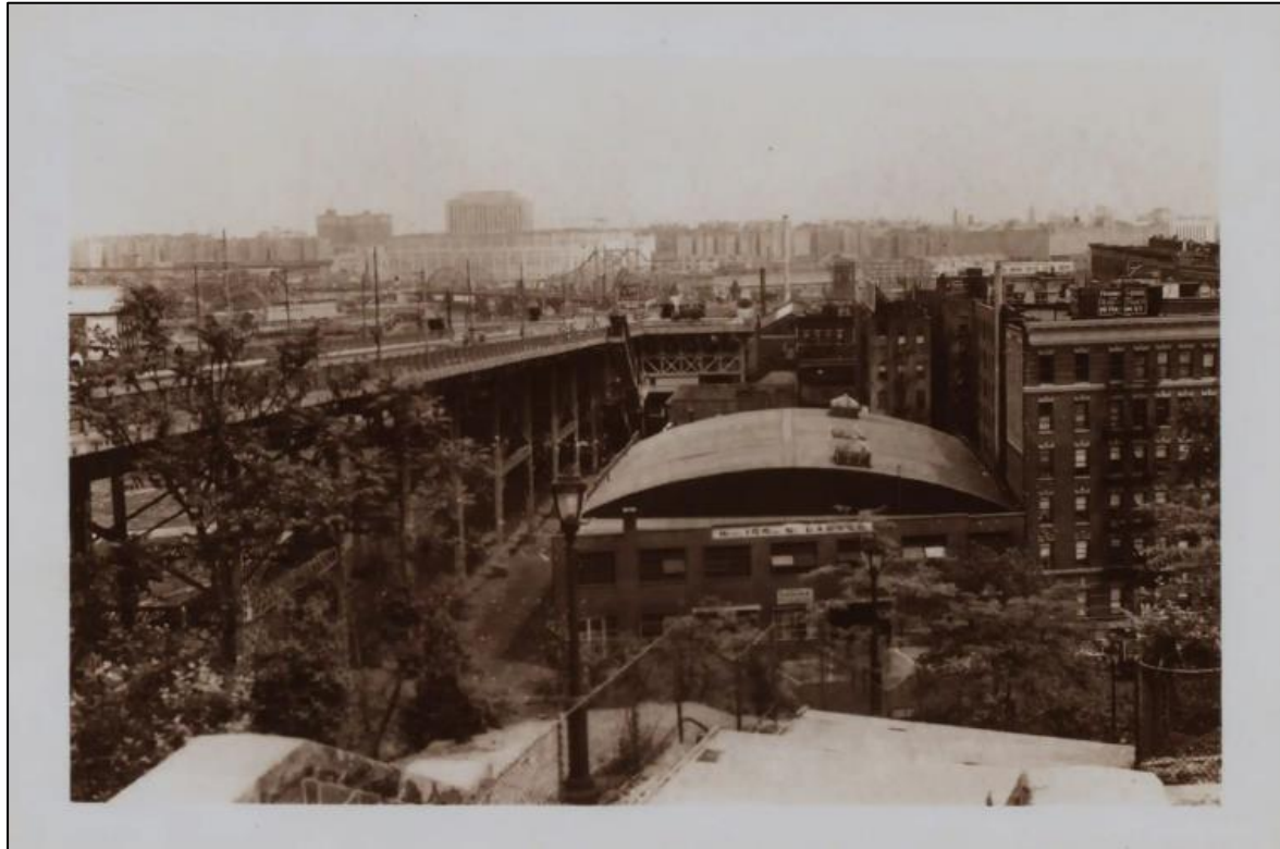
Figure 41. Eastward showing the viaduct carrying 155th Street over this point. In the background is the Bronx shore of the Harlem River. Beyond the 155th Street Bridge appears the super structures of the Yankee Stadium and the new Borough Hall Building (Recreation and Hobbies-Baseball 1940-1928).
