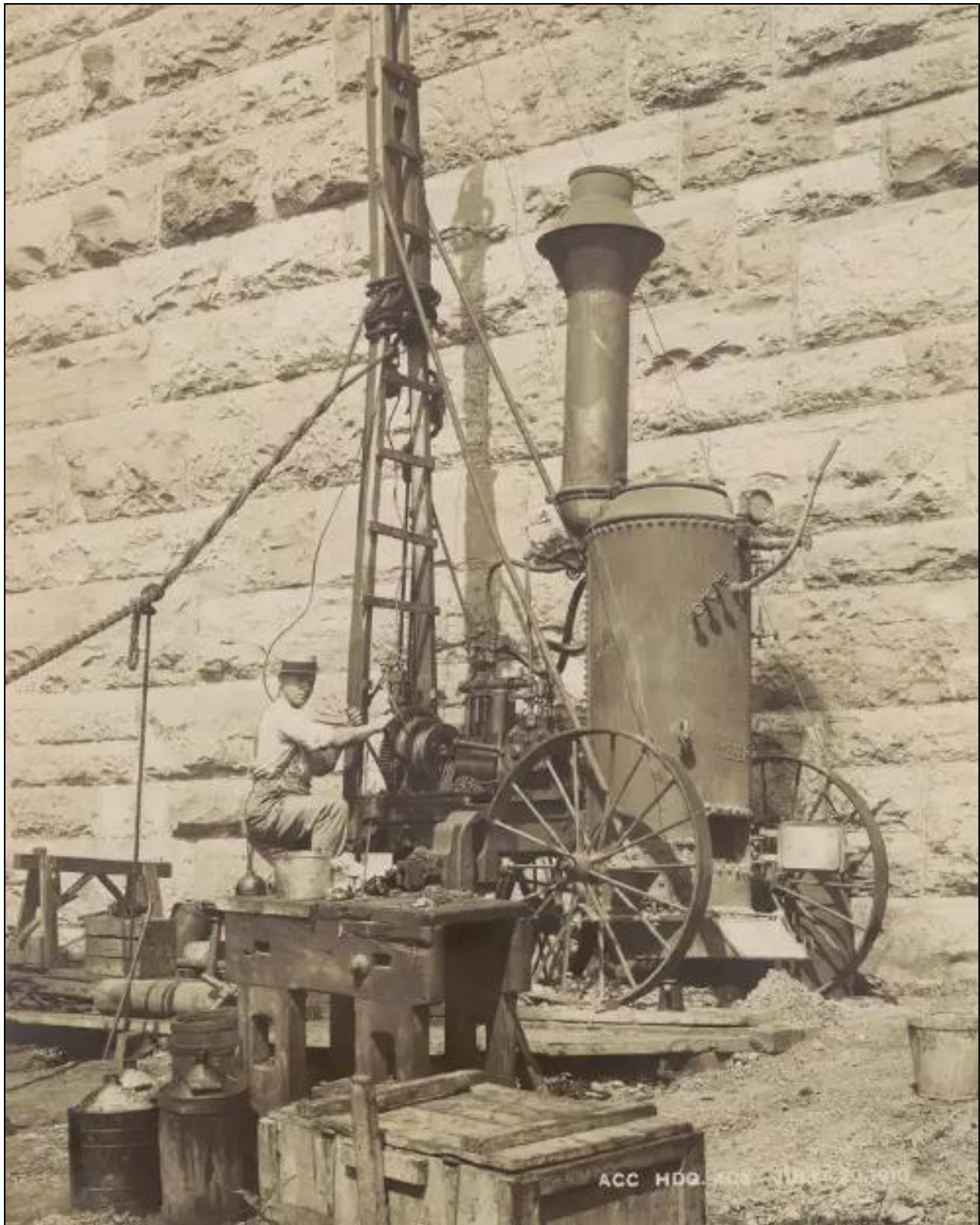
Figure 25. Board of Water Supply. City Water Tunnel No. 1. A portable drill rig collects core samples of the rock deep below upper Manhattan. These borings helped geologists and engineers to determine the best route for the 18-mile City Water Tunnel No. 1. The rig is set up near 156th Street and the Harlem River Speedway, originally built for horse racing and replaced by Harlem River Drive in 1964. July 20, 1910 (Urban Archive, Board of Water Supply).
