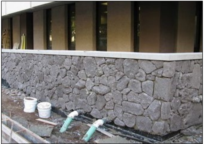
Figure 33: Dry floodproofing in the Midwest.
