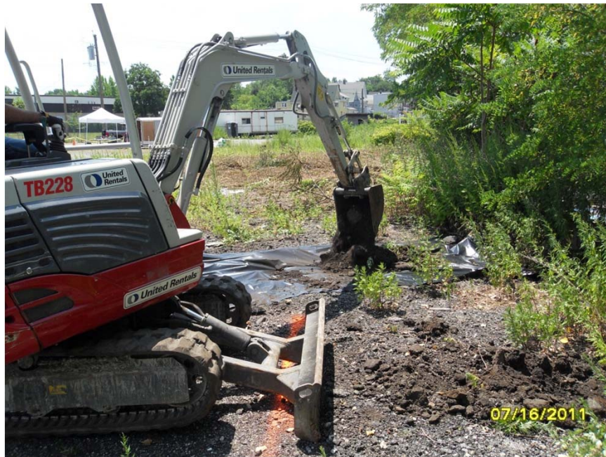
View of test pit excavation
