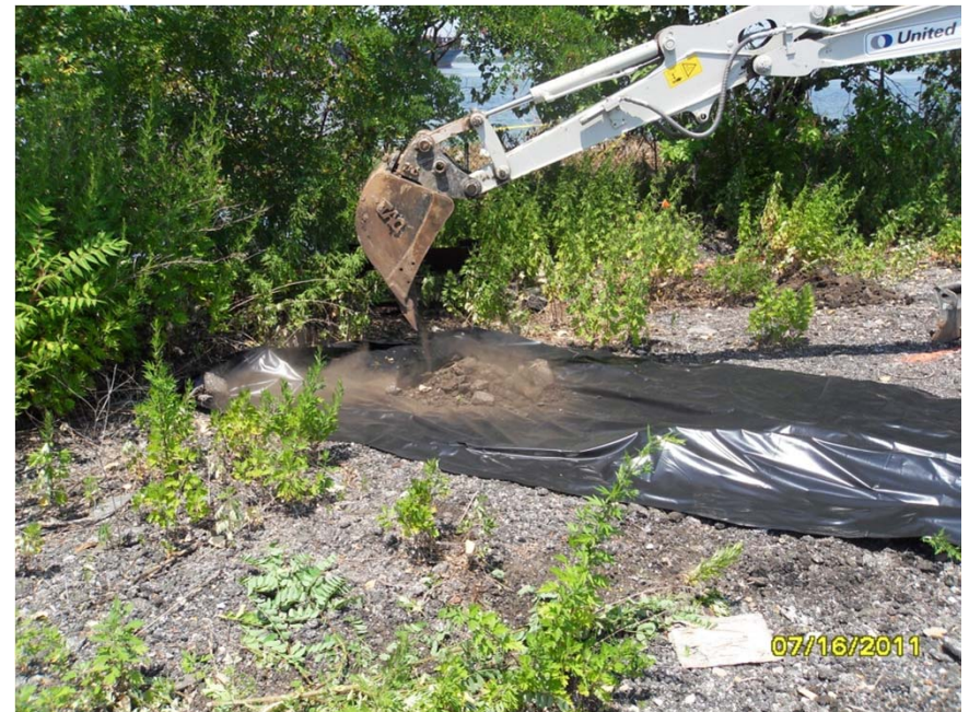
View of test pit excavation
