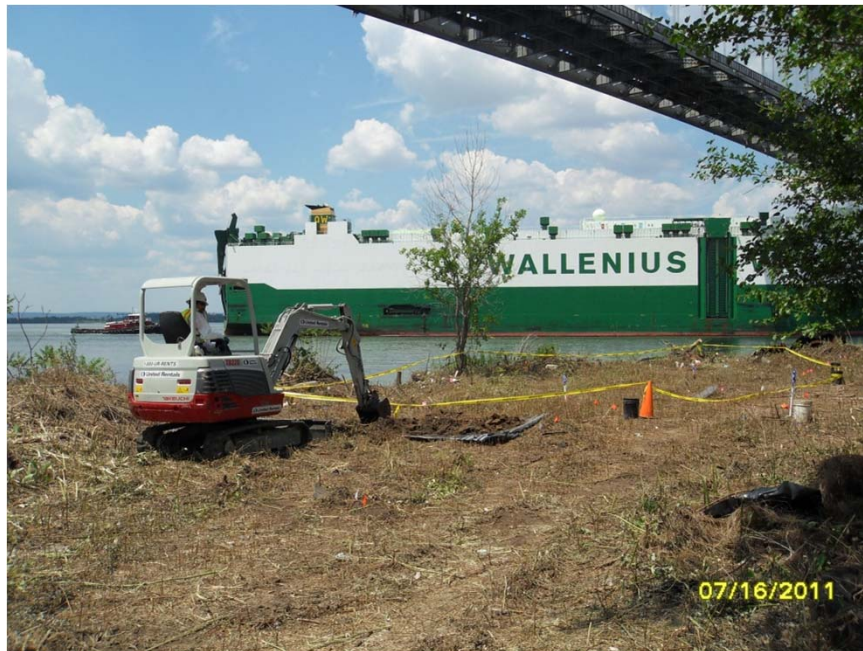
View of test pit excavation
