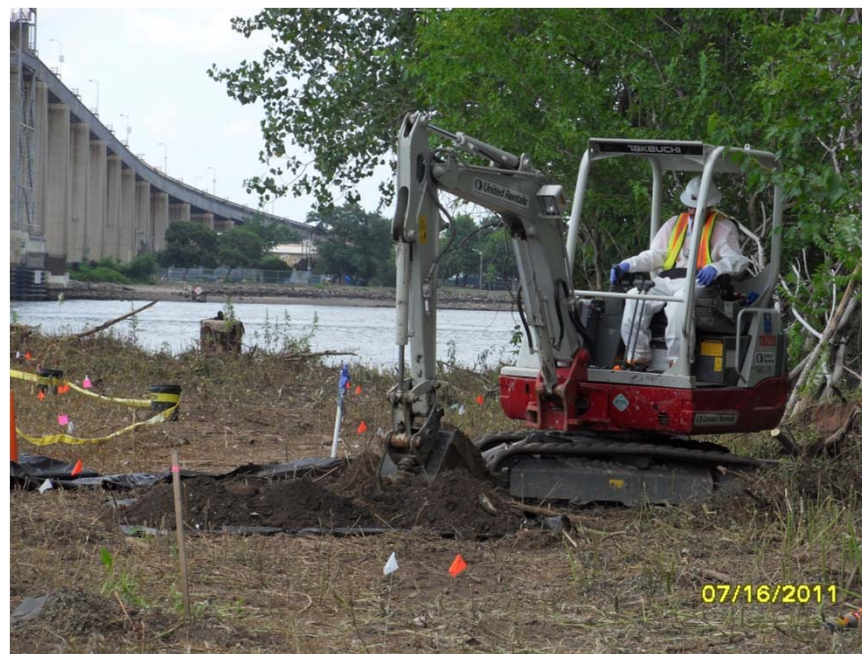
View of Test Pit excavation
