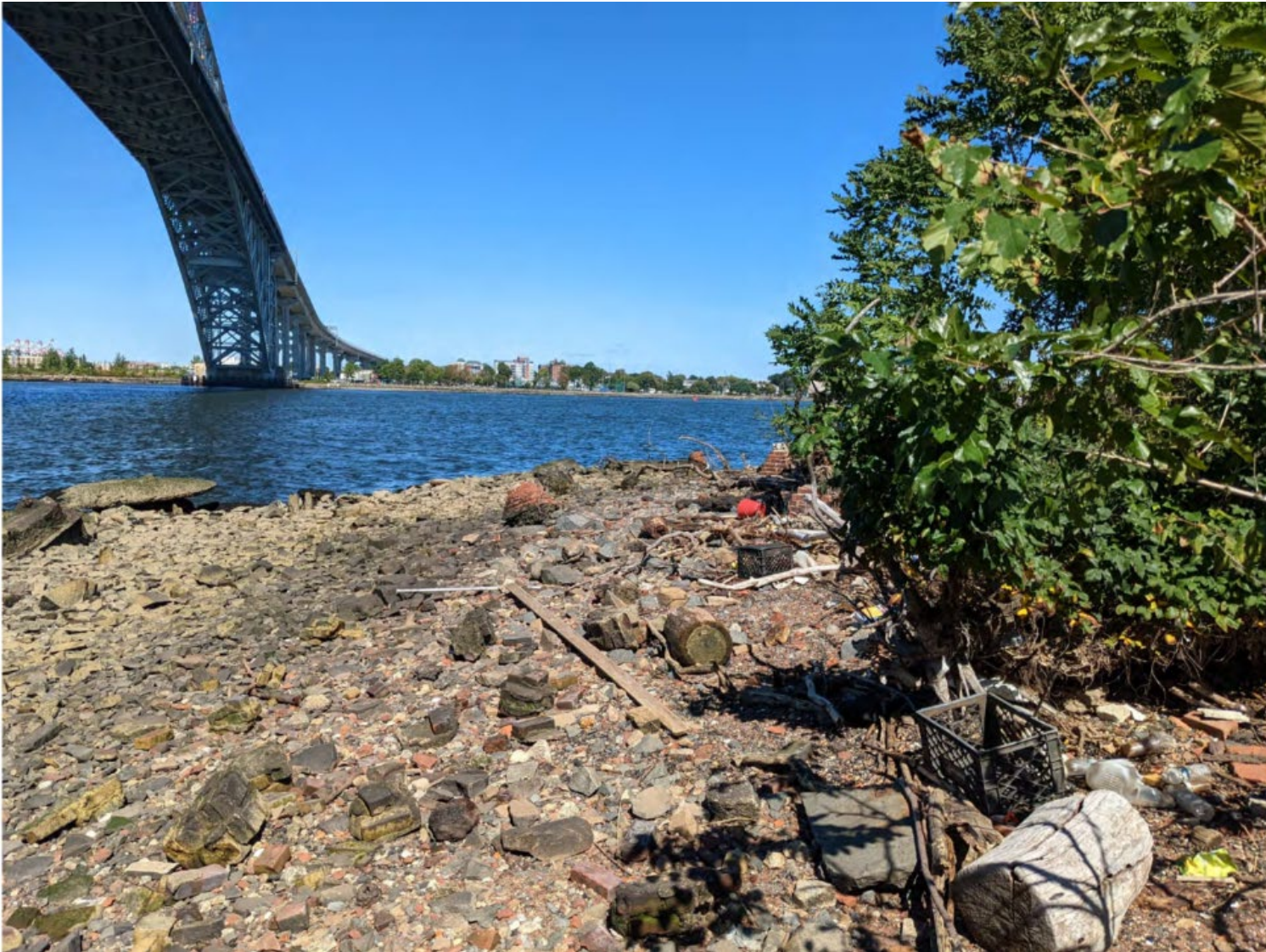
Figure 3 – Site Photograph, Rocky Kill Van Kull Shoreline (facing north)
