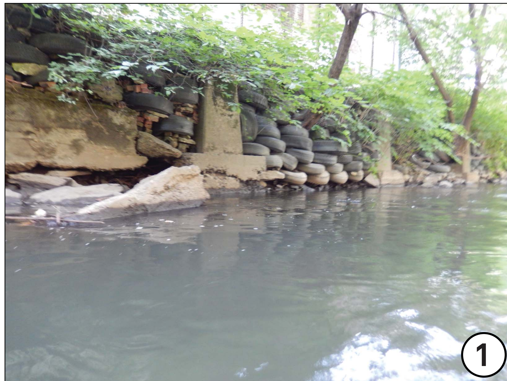
21 Jul 2014: Concrete/tire wall, downstream east bank
