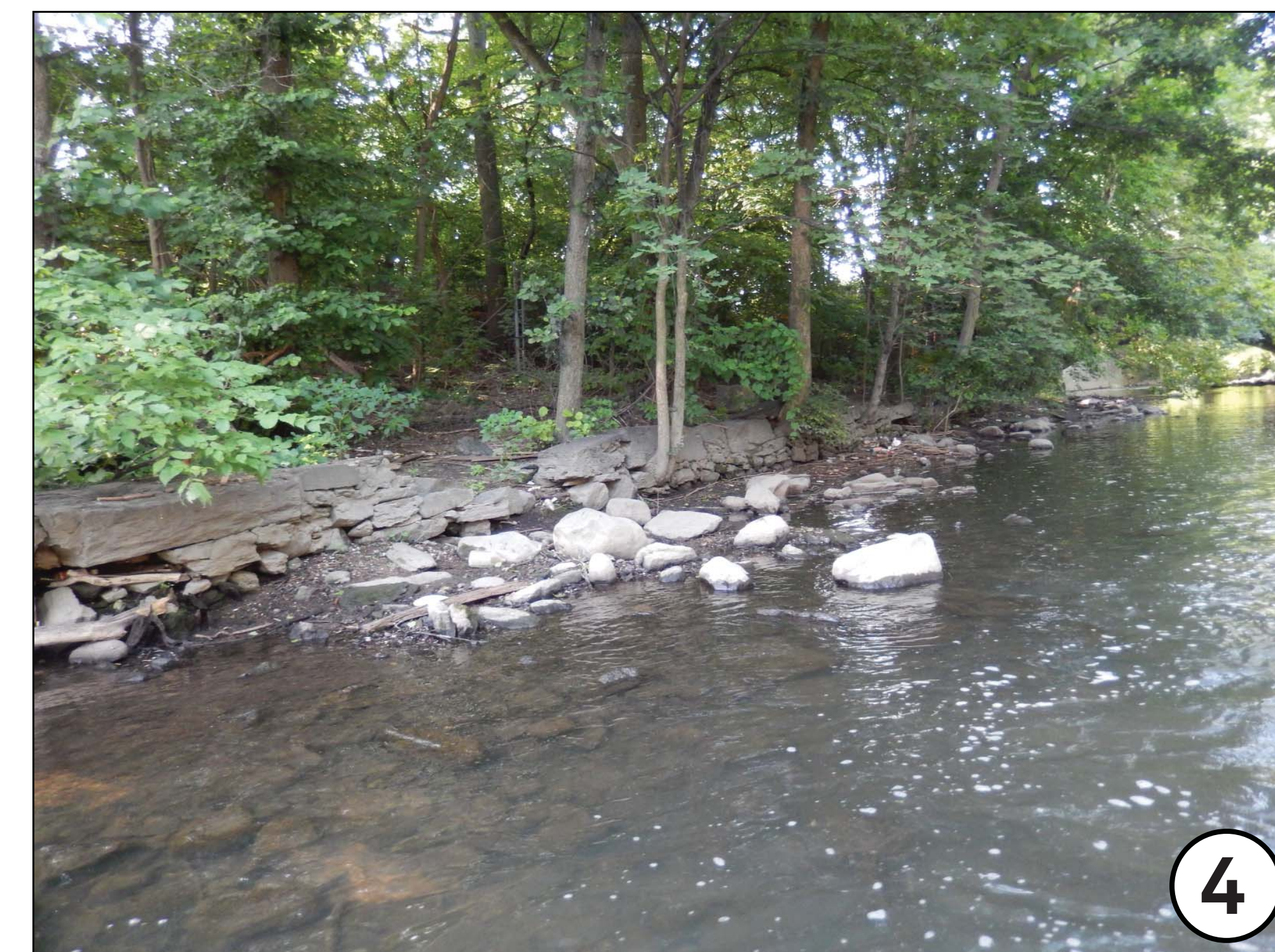
21 Jul 2014: Dilapidated armoring, upstream east bank
