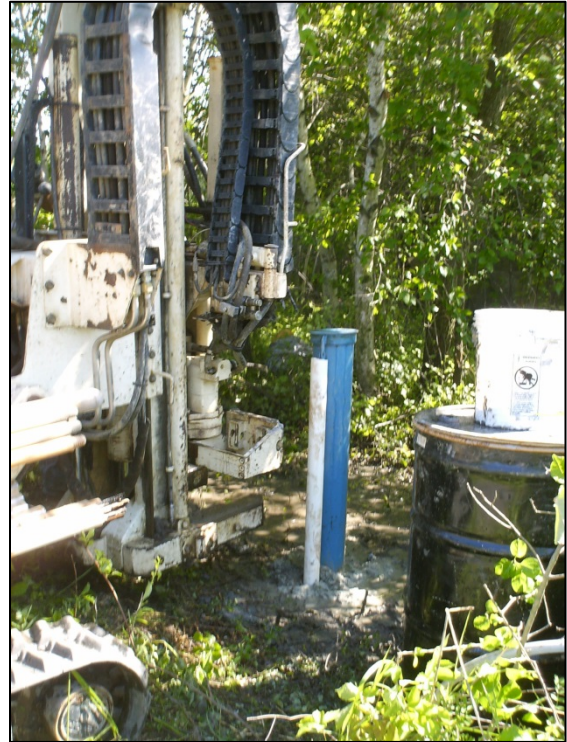
Figure 5 - Installation of a well at the former Raritan Arsenal for groundwater characterization.
