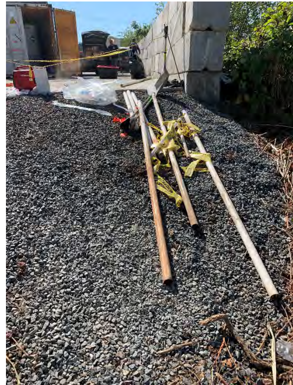
PVC pipe removed from soil borings
