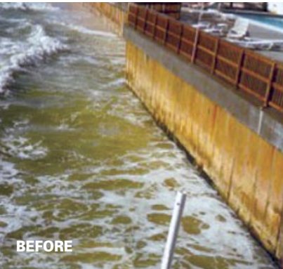
Beach nourishment, which adds sand to the coastal system, protects people and property from the effects of hurricanes and coastal storms by widening a beach and advancing the shoreline seaward. This project was constructed at Panama City Beach, Fla.
