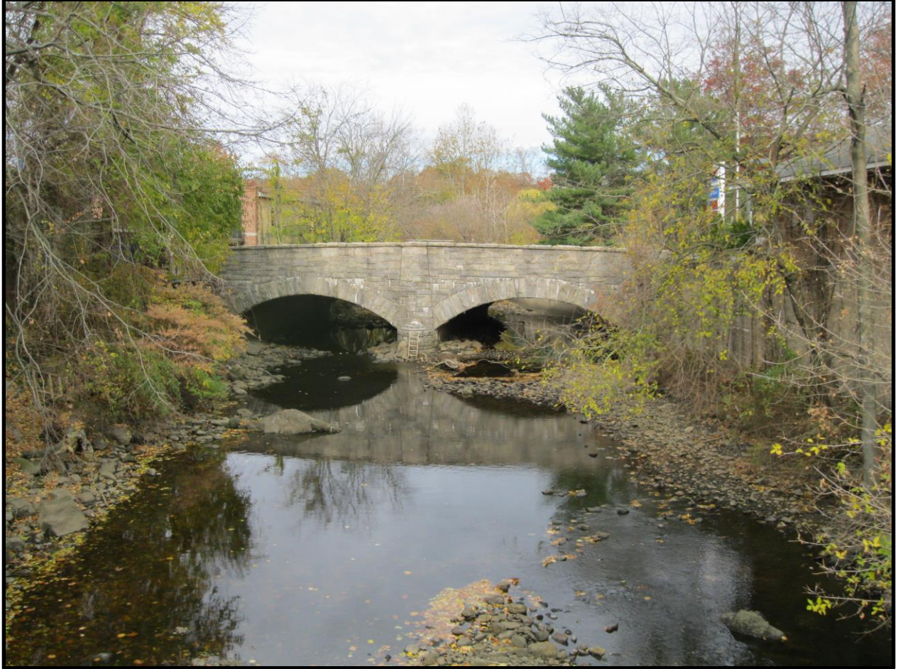
The west bound lanes (Hillside Avenue) of the Route 1 Avenue Bridge (2015)
