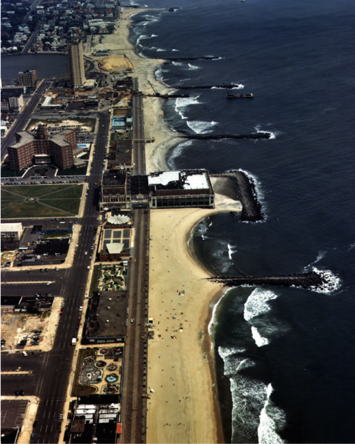
Figure 1-5. Oblique aerial photograph of pre-construction beaches at Asbury Park looking north.
