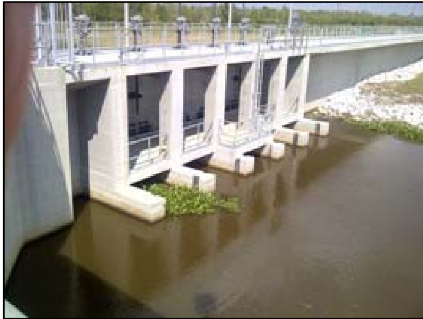
Figure 28: Sluice Gates with Box Culverts Closure
