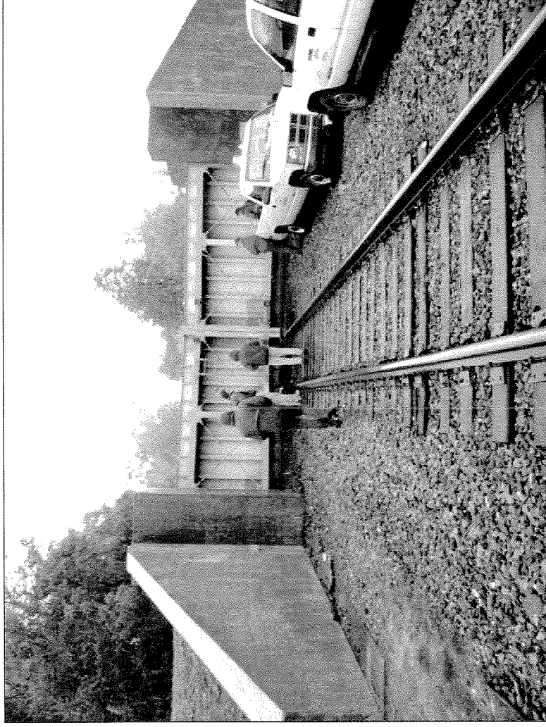
Railroad Closure Structure, Lockhaven, PA. Gates in closed position. The height above railroad grade of the completed closure structure and levee across the NJ Transit tracks will be similar to the height of the levee and walls of the Lockhaven structure.
