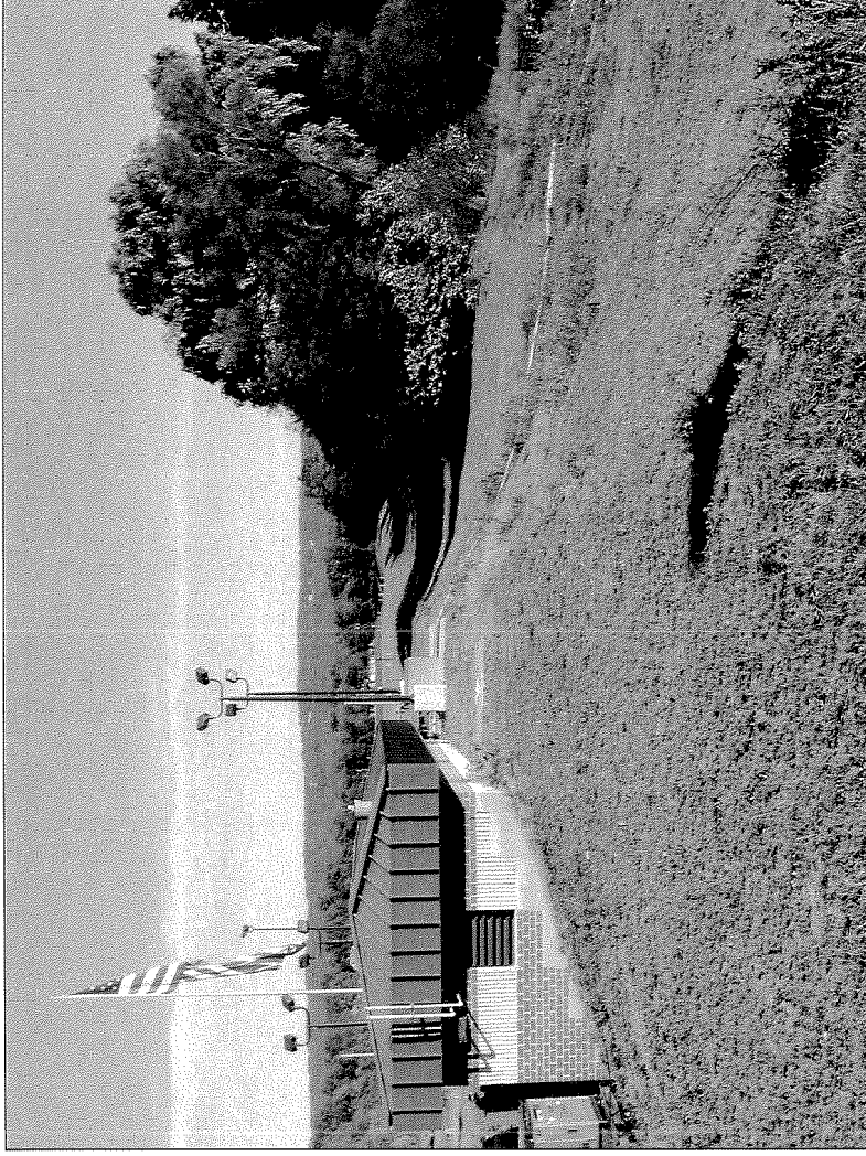
Bound Brook: The Segment T pump station is built into the Segment T levee. The pump station on Segment R-2 will also be built into the levee, however, the R-2 pump house will run for a greater length along the levee as a small meeting/locker room will be included in its design. Photo: April 2007.
