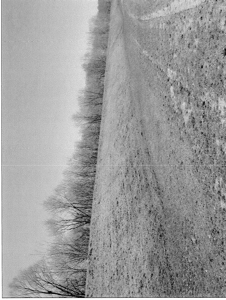
Bound Brook: Segment R-1 Levee in the vicinity of Tea Street, north of Talmage Ave. This is a typical view of a completed levee. The R-1 levee near its intersection with the railroad track crossing will be similar in height. The R-2 levee, near to the historic railroad bridges will be approximately 5 feet higher. View looking northwest, April 2007.
