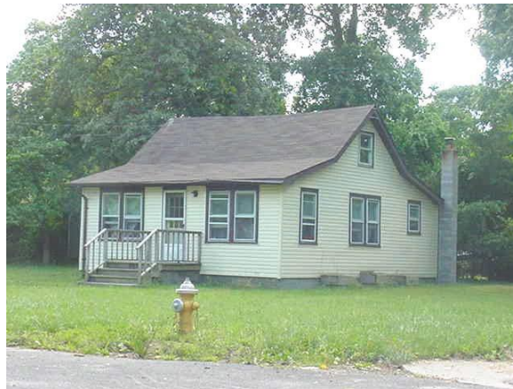
Figure 3: Typical Raised (Crawlspace) Foundation Type
