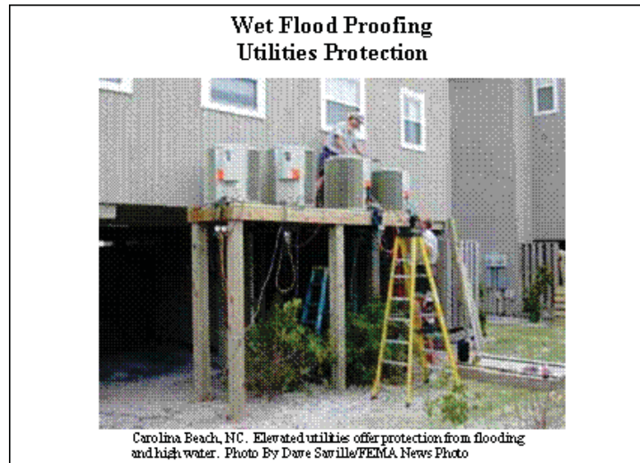
Figure 12: Wet Flood Proofing Utilities Protection
