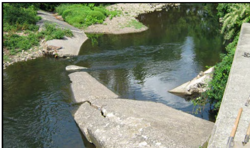
Figure 5: The concrete weir that helped channel water into the Little Falls Laundry. The central part of the weir was washed out during Hurricane Irene, after this picture was taken (Hartgen Archeological Associated 2013).
