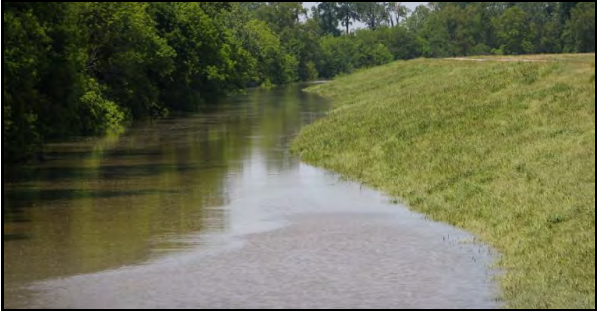
Figure A-3. Example of a levee holding back flood waters.
