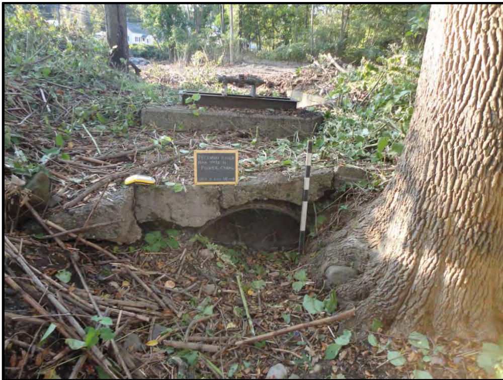
Figure 7: The downstream side of the Little Falls Laundry headrace sluice gate and steel culvert (Hartgen Archeological Associates 2013).
