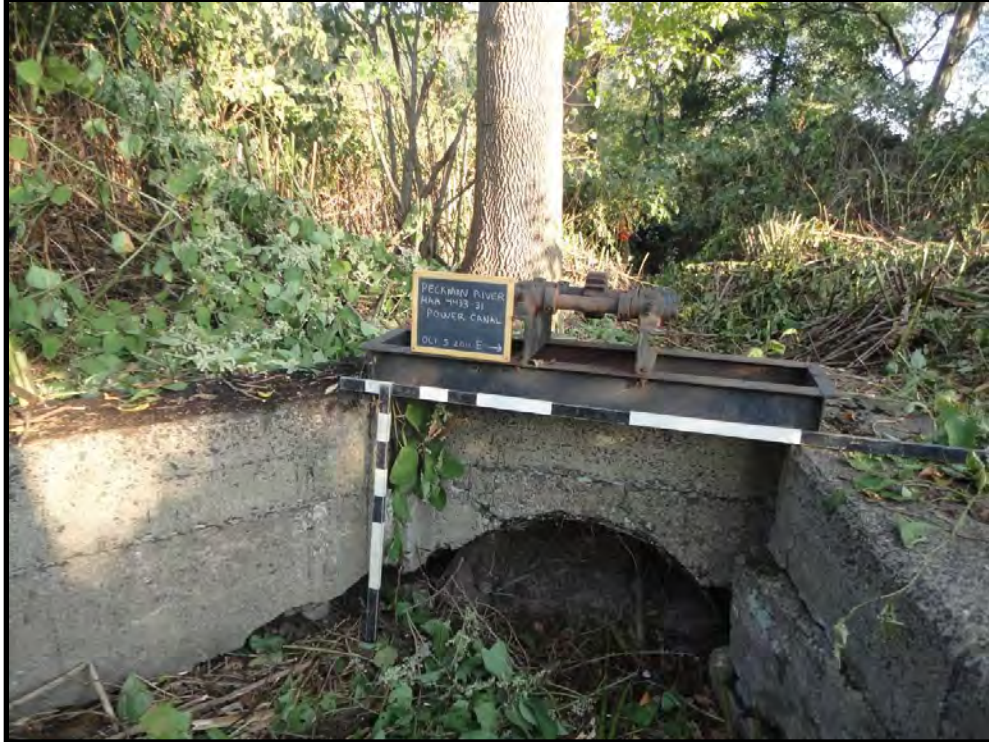
Figure 6: The Little Falls Laundry headrace's sluice gate and steel culvert (Hartgen Archeological Associates 2013).
