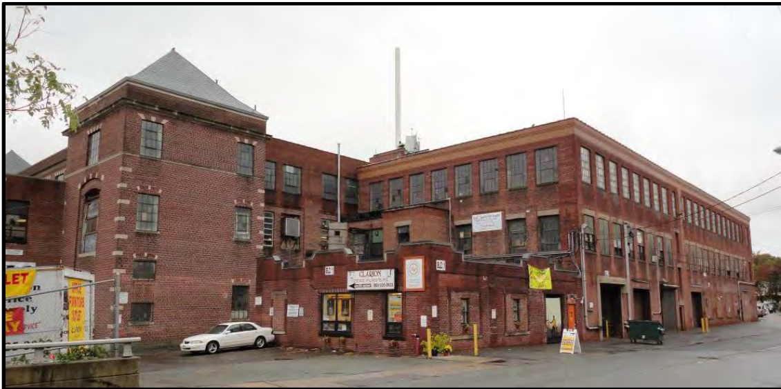
Figure 4: The Little Falls Laundry, 101 East Main Street (Hartgen Archeological Associates 2013)
