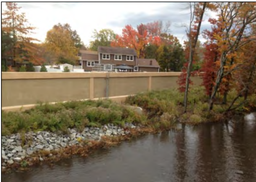
Figure A-4. An example of a permanent floodwall in Middlesex, New Jersey.
