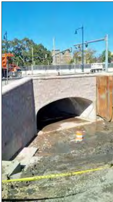
Figure A-2. Example of a culvert similar in size to the proposed Peckman River diversion culvert.
