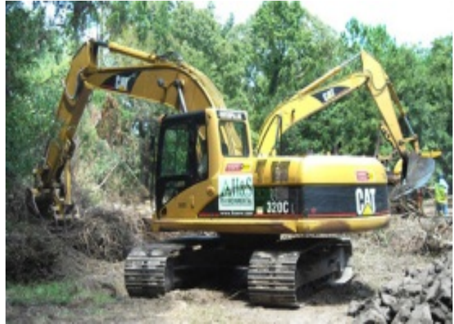
Site preparation and excavation activities. (File Photo)
