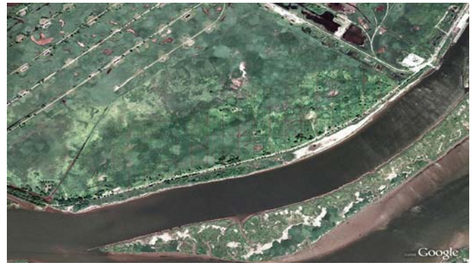
Aerial shot of Area 12 - Former Raritan Arsenal – Edison, New Jersey
