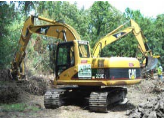
Site preparation and excavation activities. (File Photo)
