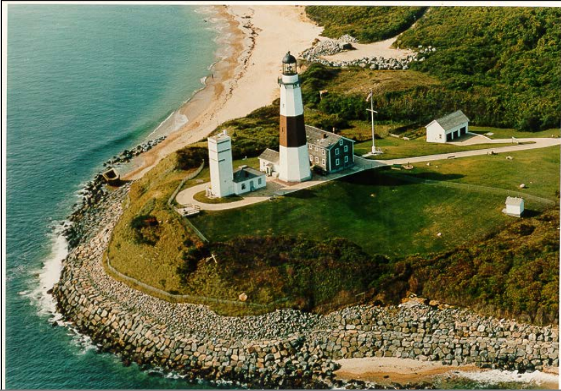
The cooperative effort of the U.S. Army Corps of Engineers, U.S. Coast Guard, New York State Department of Environmental Conservation, Long Island Office of Parks, Recreation and Historic Preservation and the Montauk Historical Society have improved the erosion control protection at Montauk Point. (c. 1995 Peter Paul Muller Jr.)
