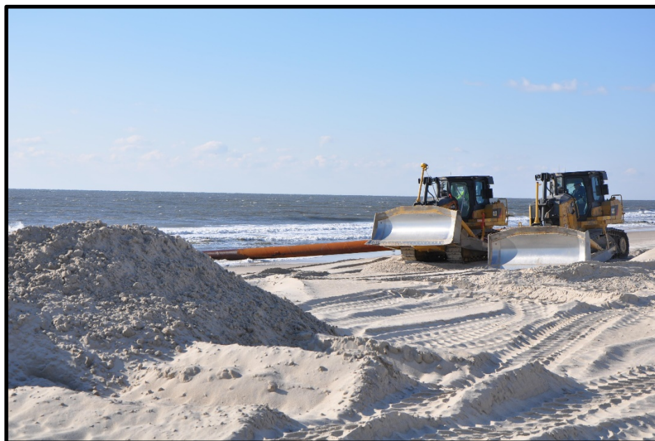
Bulldozers move sand for a USACE CSRMR project in Westhampton, NY.
