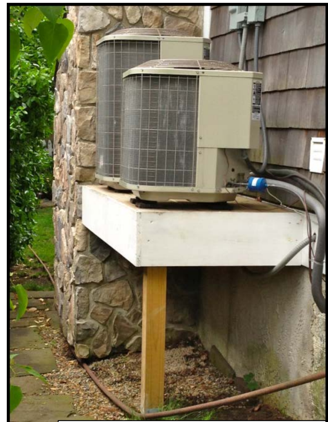
Wet Floodproofing
