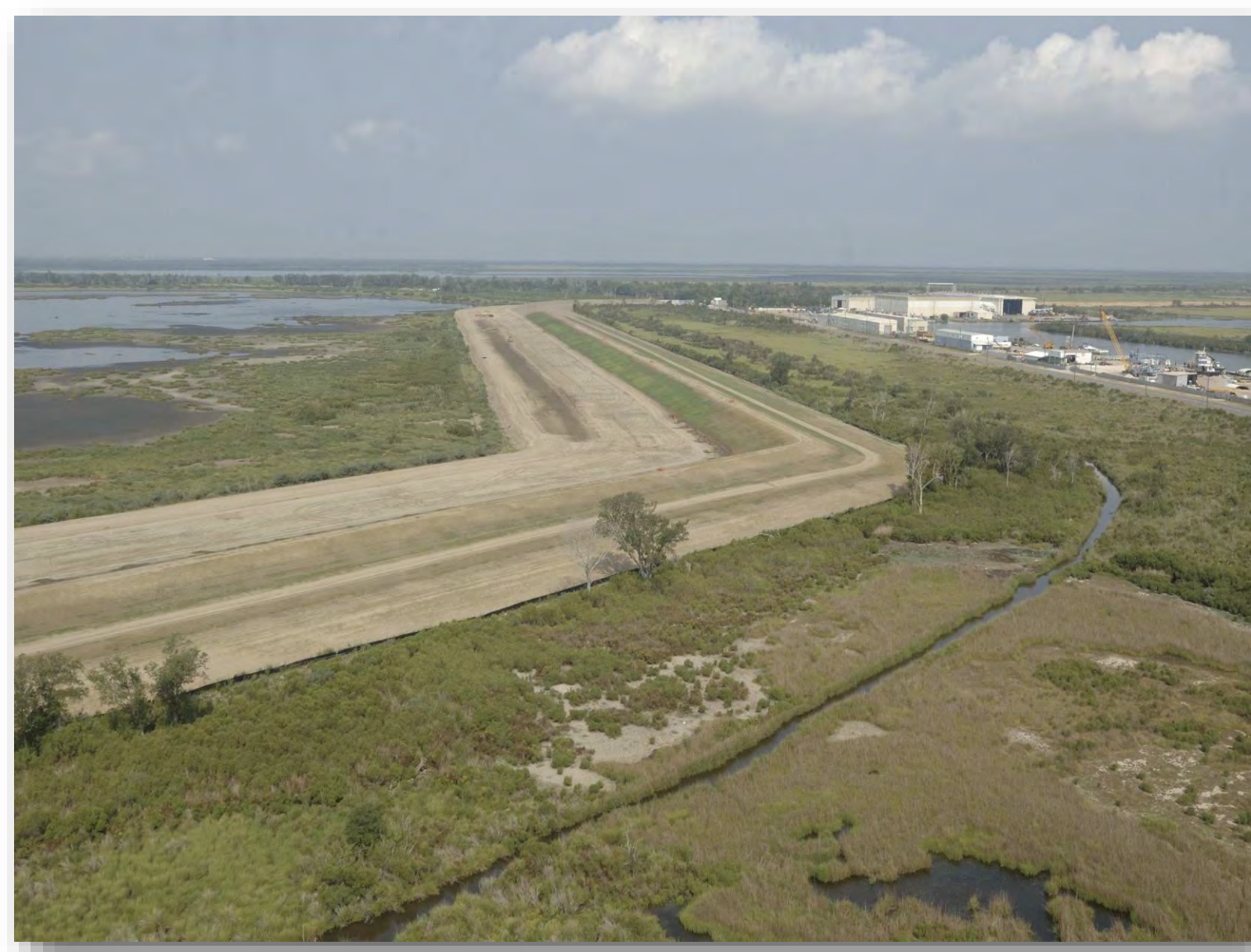
Levee – New Orleans, LA
