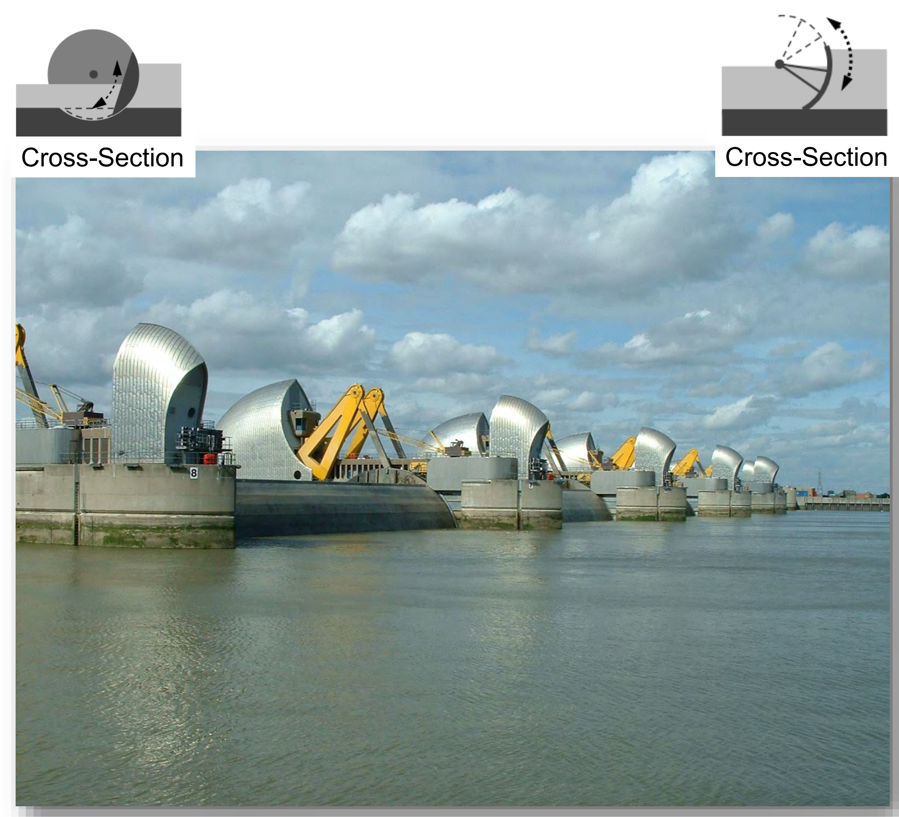
Thames Barrier – London, UK Rotating Sector Gate, Tainter Gate
