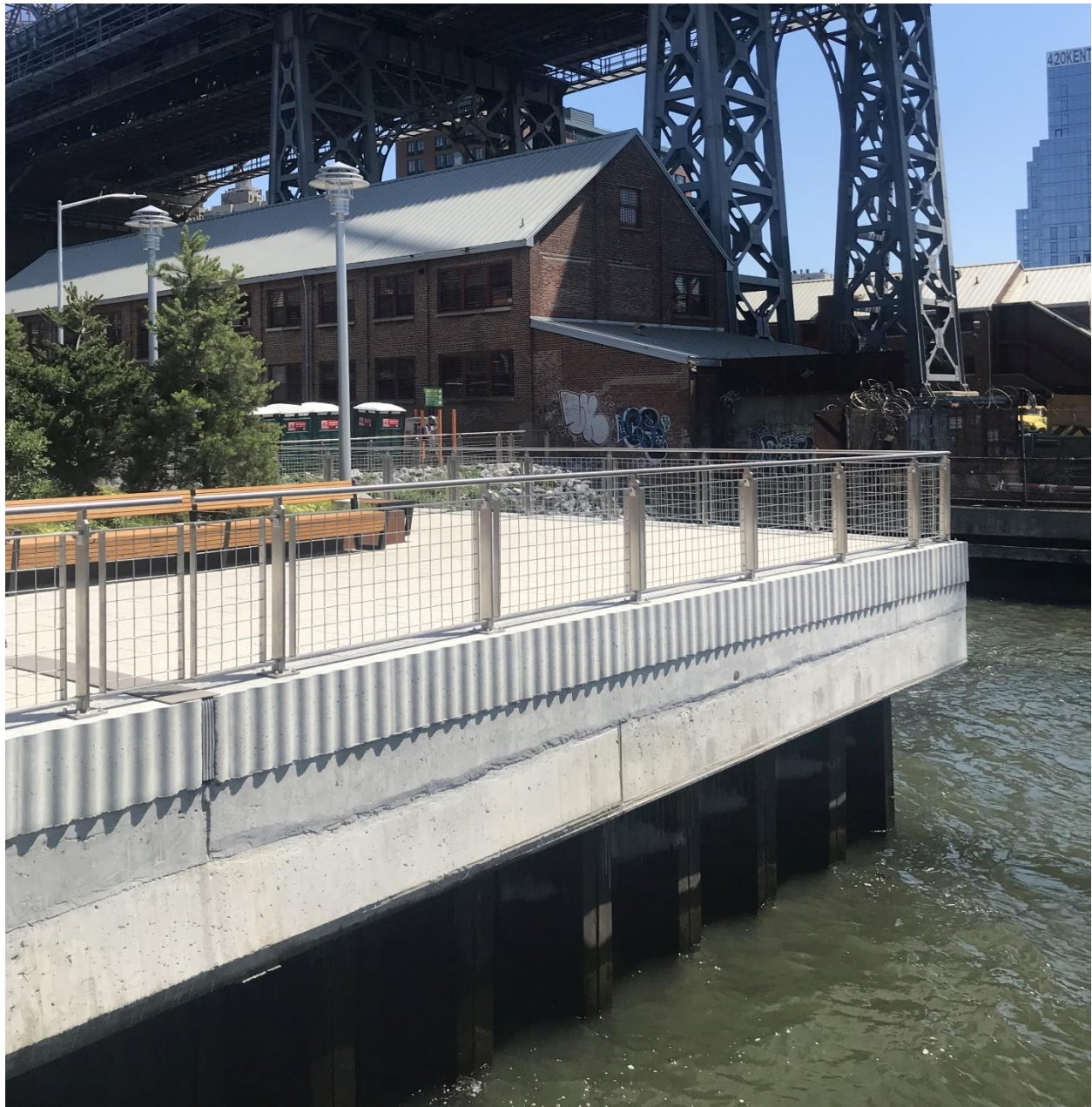
Figure 4-8: Bulkhead at South 5 th Street Brooklyn, NY
