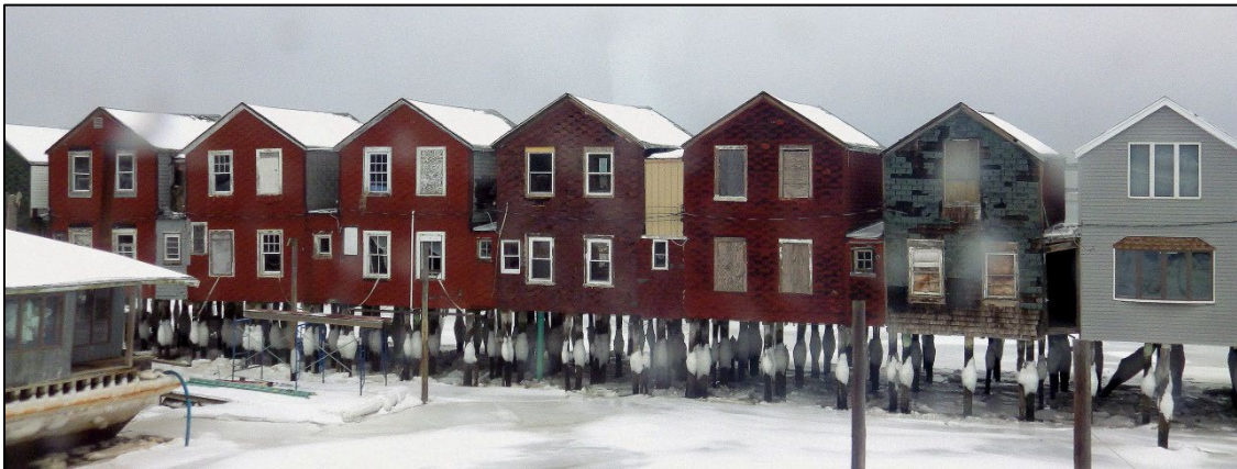
Figure 15: Photographs of the eligible properties near the Hammels high-frequency flood risk reduction: New York City Transit System building (top), 2 Beach 85 th Street (middle) and the Hammels Pier (bottom) (NYSHPO CRIS 2019).
