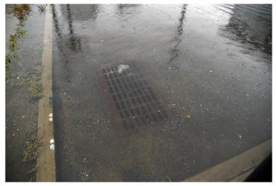
Figure 4-1: Spring High Tide Flooding of Storm Drain
