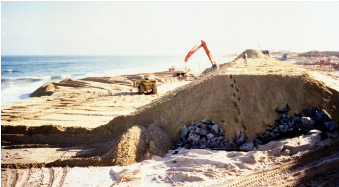
Figure 7-12: Buried Seawall Example at Dam Neck, Virginia (USACE, 1999)
