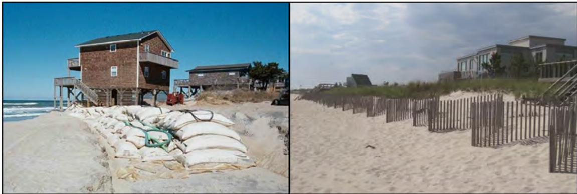
Figure 17: Example Applications of Geotextile Sand Containers
