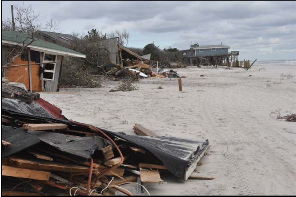
Figure 4: Post-Hurricane Sandy Photo at Davis Park
