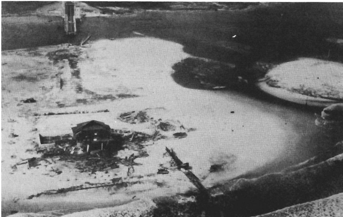
Figure 2-5. Conditions in the area of Westhampton Beach after the Hurricane of 1938. Damages shown in the photo include significant damages to the west bay bridge, and a breach of the barrier island to the east of the bridge.
