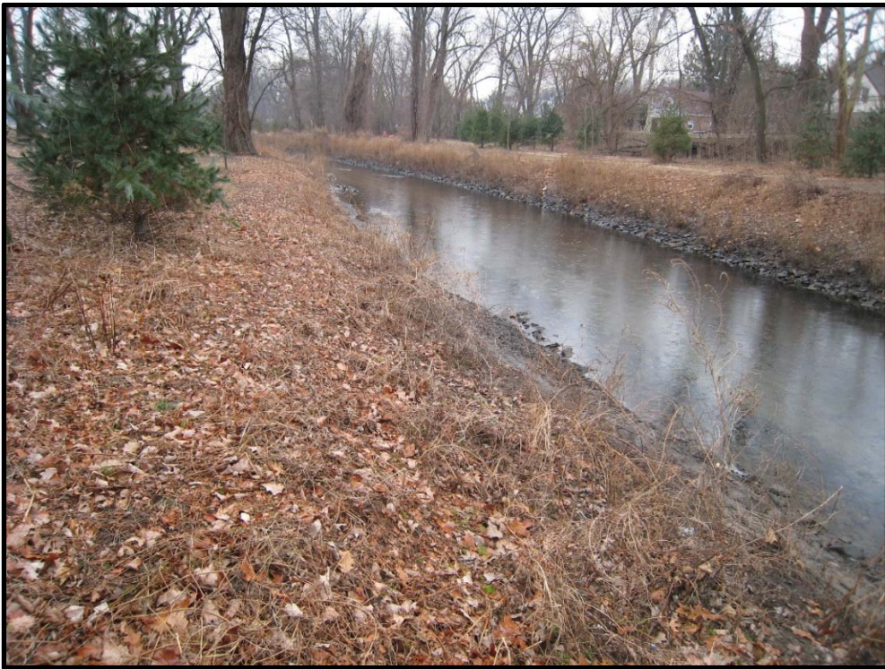
Figure 49: Example of a Sloped Grassed Bank or Trapezoidal Channel in Winter.
