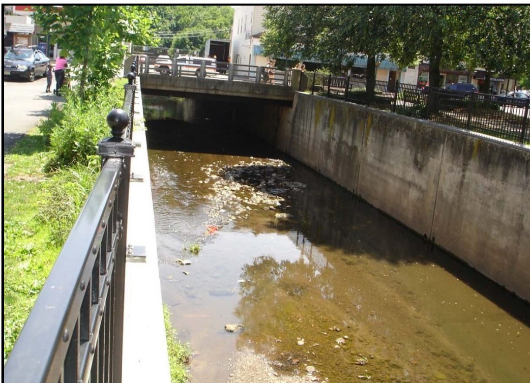
Figure 46: Example of Concrete Retaining Walls: Sheldrake River East of Mamaroneck Avenue.
