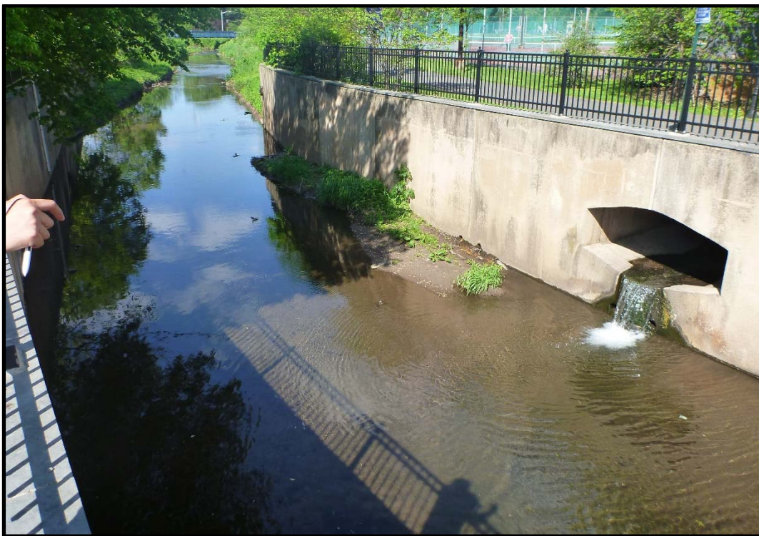
Figure 45: Example of Culvert Structure
