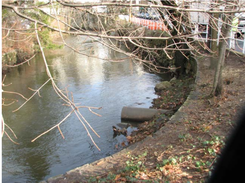
Bronx River facing north, southern portion of the site
