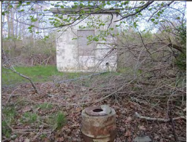
Bldg 2010 and well head Pb in soil
