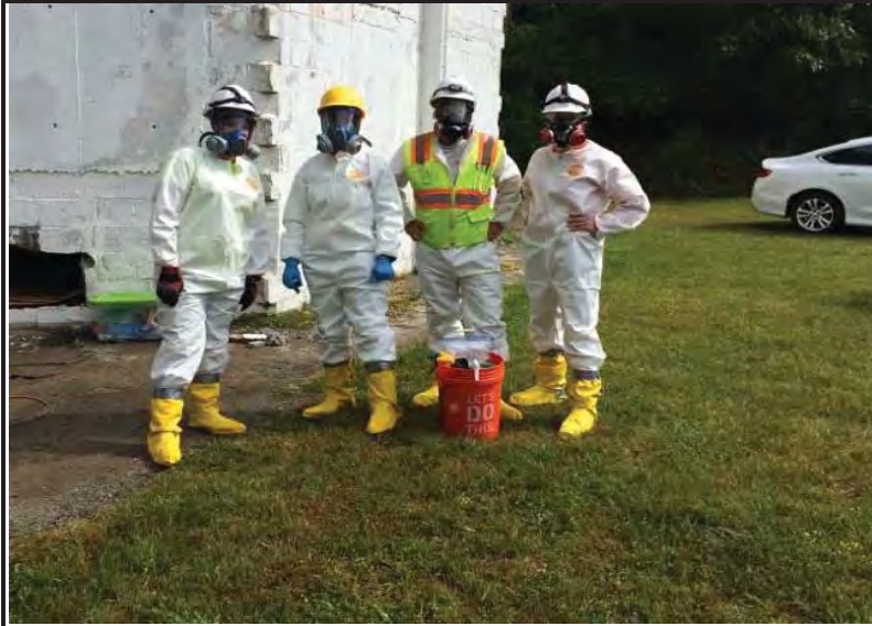
Photo 3. The team in safety gear before entering Battery 113.
