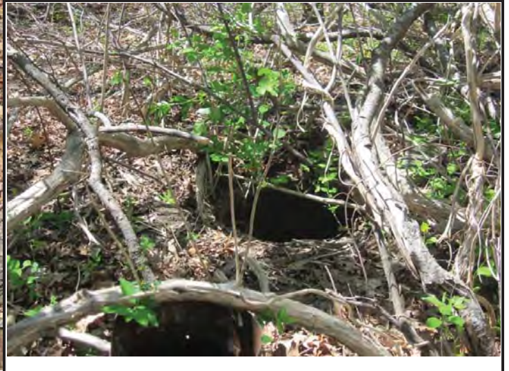
Open manhole (old cesspool) at suspected tank F (not found)
