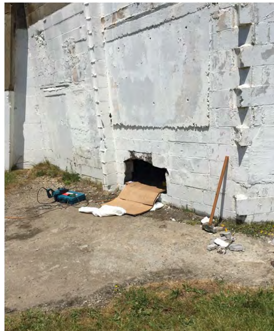
Battery 113. Final crawlspace entrance to Battery 113, June 2016.
