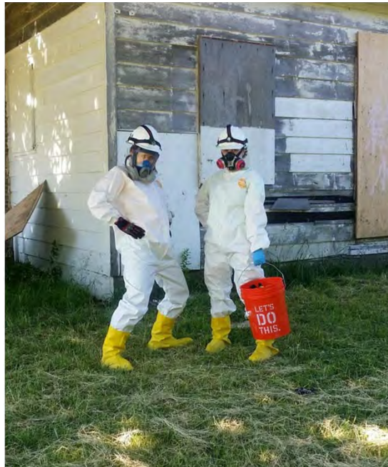
Building 107 (Electrical Substation). Greta White and Amanda Martin (AECOM) in PPE before entering Building 107 to collect concrete chip samples for PCBs, June 2016.
