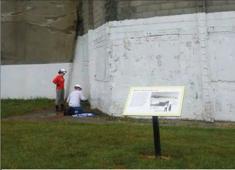
Photo 1. Demolition of Battery 113 entrance.
