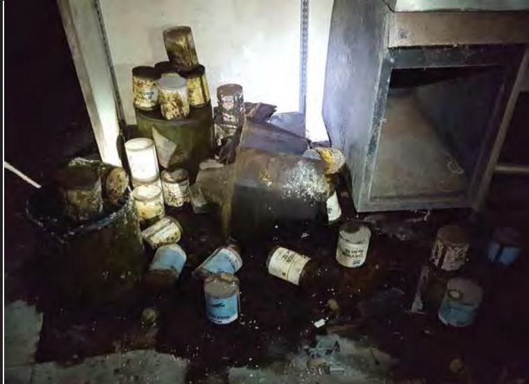
Photo 1. Miscellaneous cans in Main Room of Building 10.
