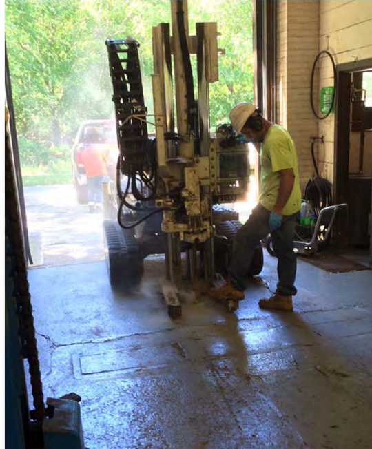
Motor Pool. Soil core collection from location MP-SB01 inside the Motor via the Direct Push 6620DT rig by Keith Precious (NEG), June 2016.
