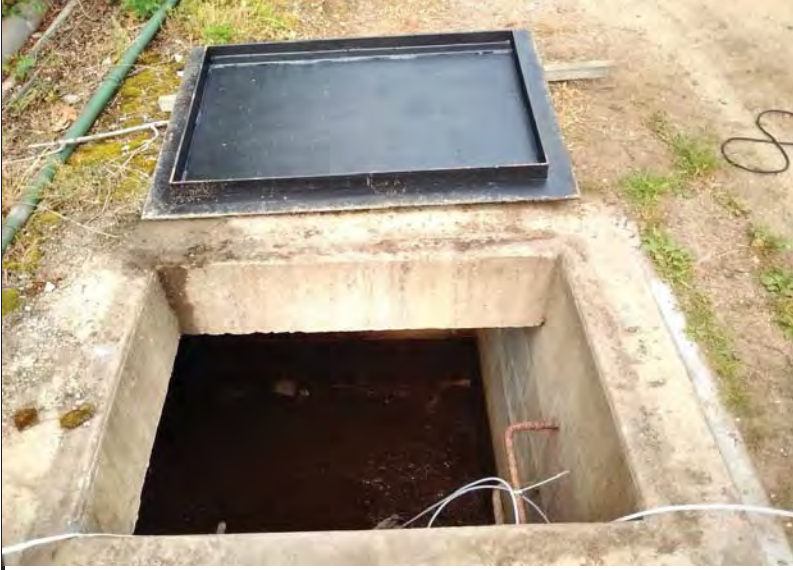
Photo 1. 3001-MW01 vault, showing confined nature of the space.
