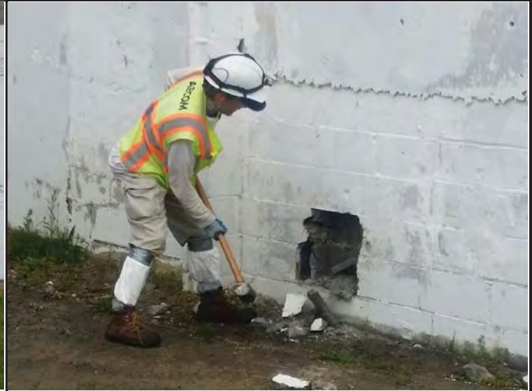
Photo 2. Demolition of Battery 113 entrance.
