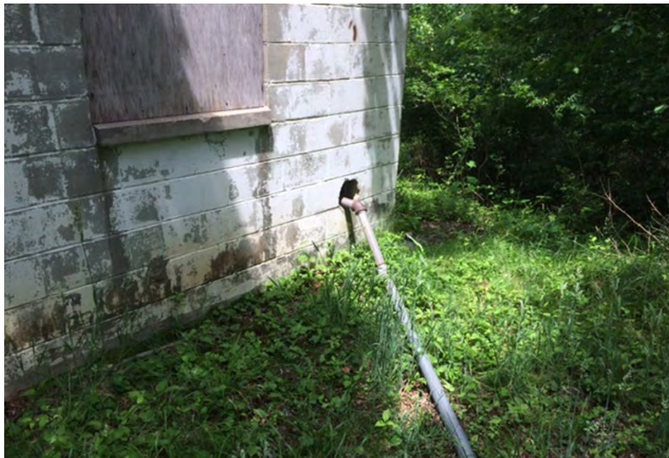
Building 2010. Pipe on the east side of Building 2010, June 2016.
