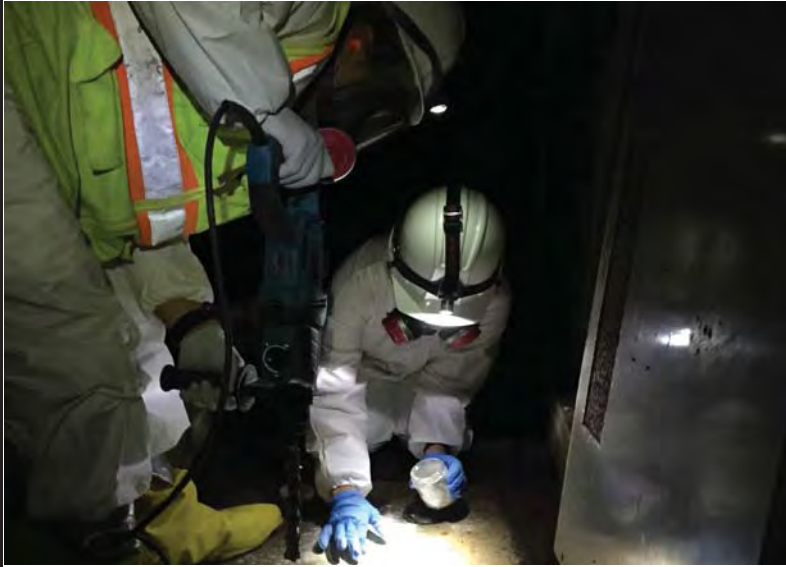
Photo 9. Concrete chip sampling with Hammer Drill in Transformer Room (Battery 113).
