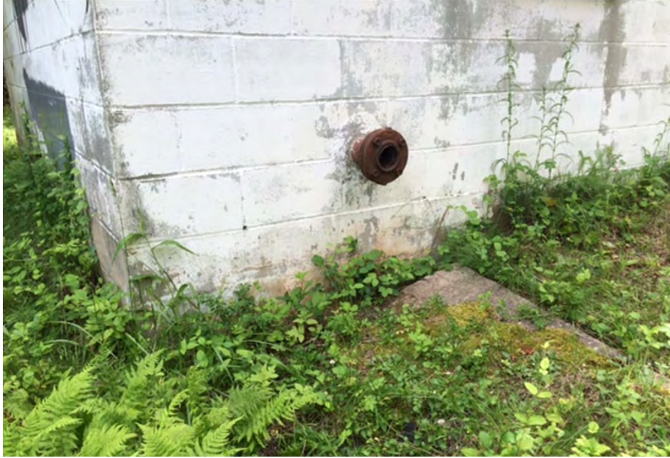
Building 2010. Pipe at Building 2010, June 2016.
