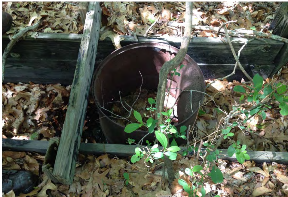
H-20. The drum at H-20, located within the wooden revetments of Camp Hero State Park, June 2016.
