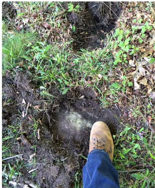
Waste Disposal System. Uncovered concrete feature/suspected septic tank or cleanout found in area to which WDS-SB06 and -SB07 were relocated, June 2016.
