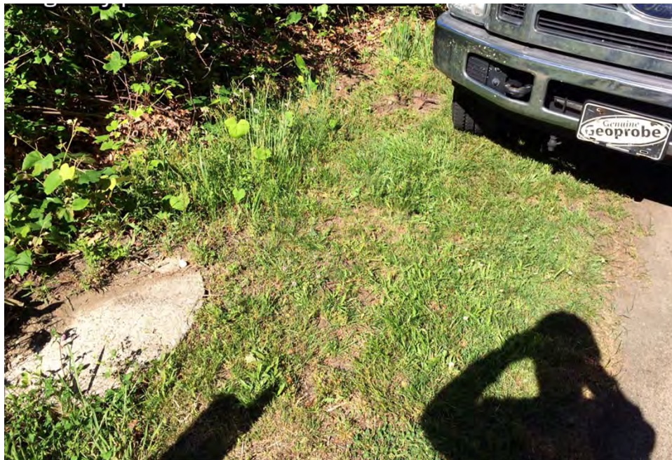
Waste Disposal System. Concrete cover/manhole near roadside at the original RI Work Plan WDS-SB06 location, June 2016.
