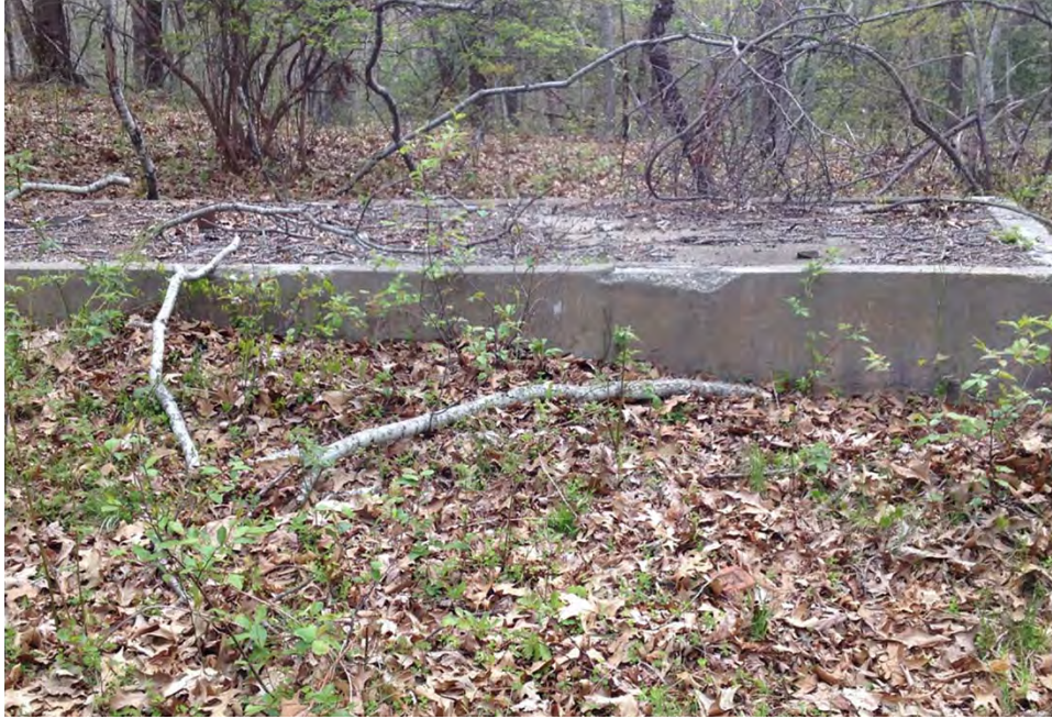
H-3. Building foundation located near H-3 identified during May 2016 site walk.
