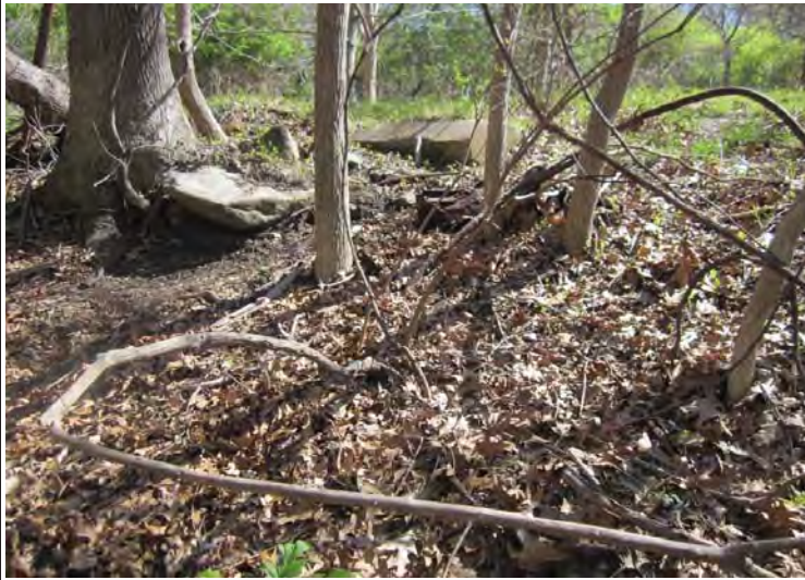
Debris at Plotting Room 113 (demolished)
