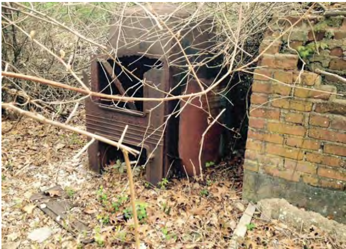
Former Building 34 debris near motor pool
