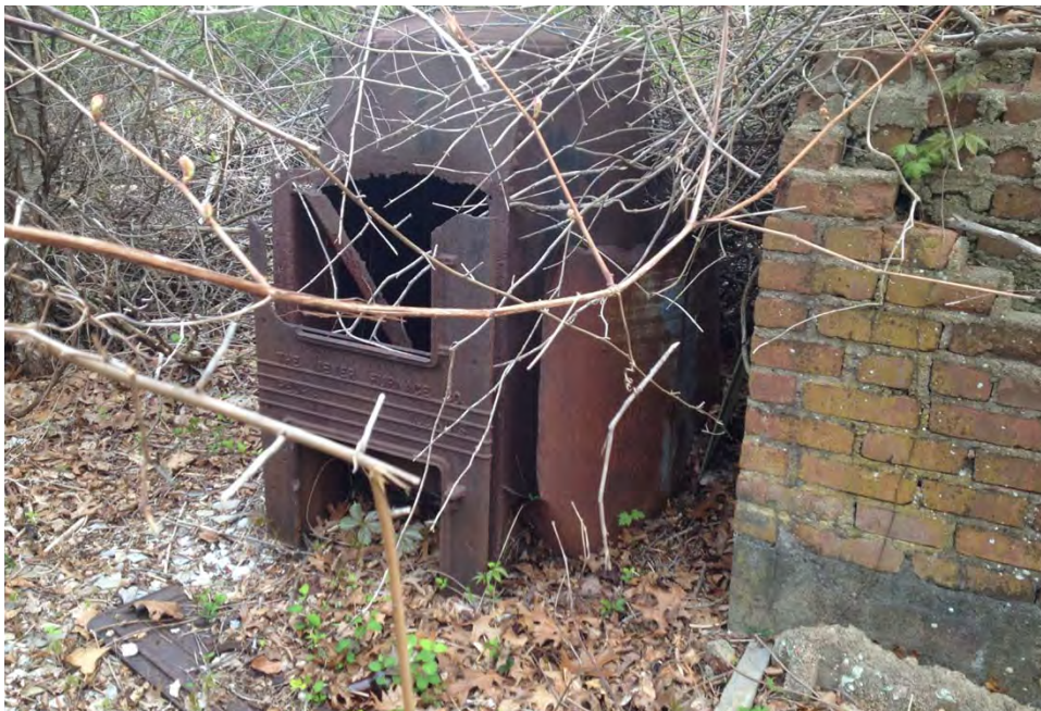
Former Building 034. Furnace at former Building 034 near former building remnants, May 2016.
