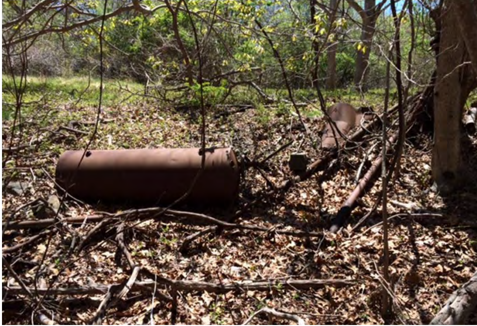
H-9. Old, rusted boiler at H-9, May 2016.
