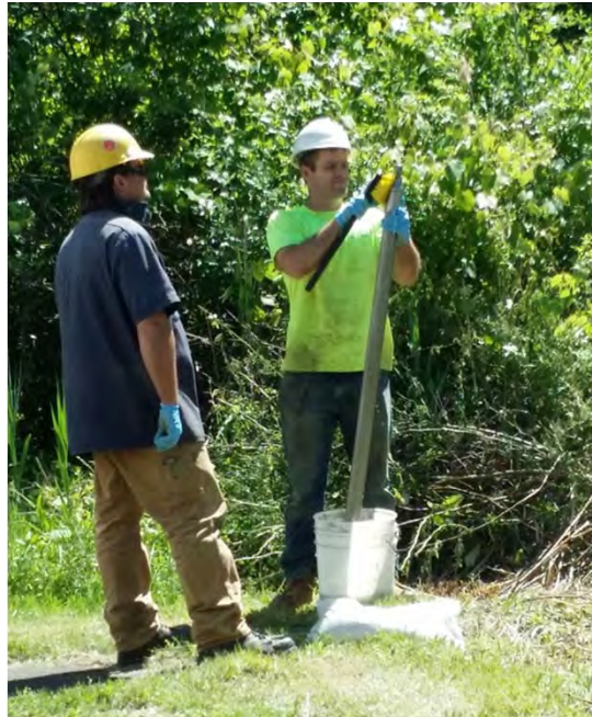
Building F100C. New England Geotech completing decontamination of the drill rod at Building F100C, June 2016.
