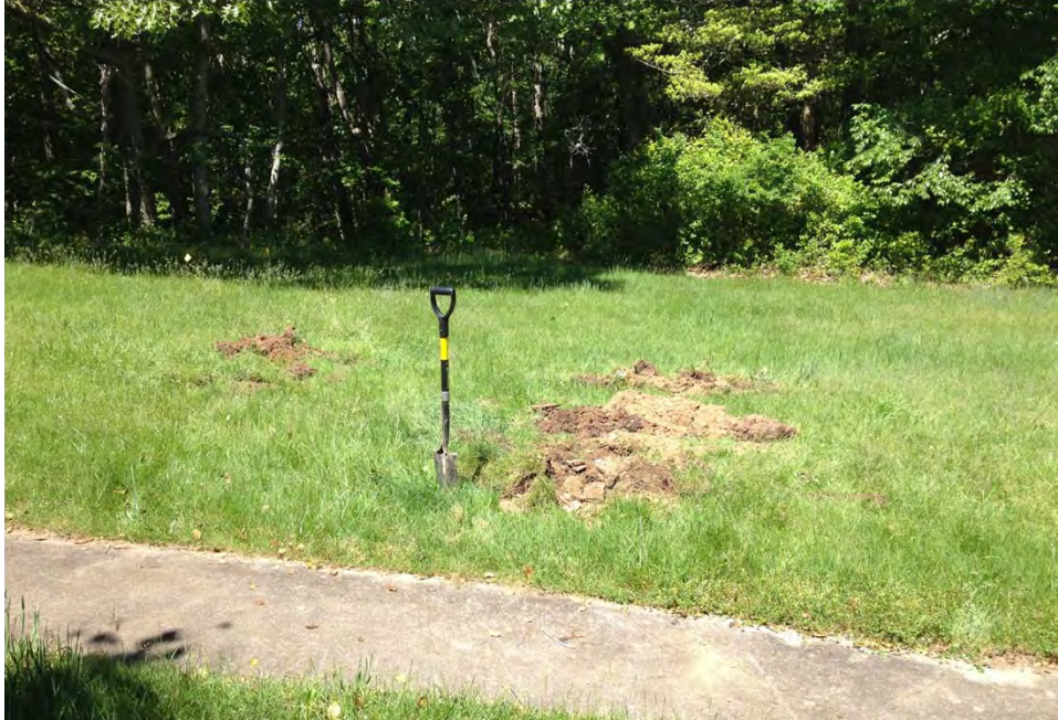
Suspected Tank C (former Building 2). "Test holes" were conducted in June 2016, to investigate anomalies identified in the May 2016 geophysical survey.
