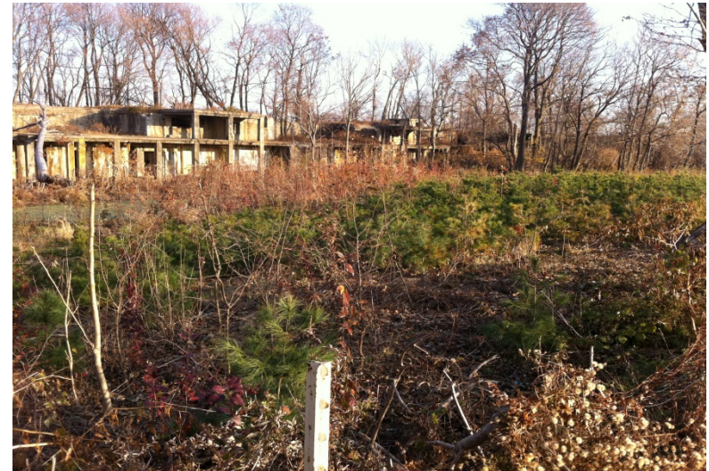
Figure 4 – Area 1, View North Towards Ft. Totten Fortifications
