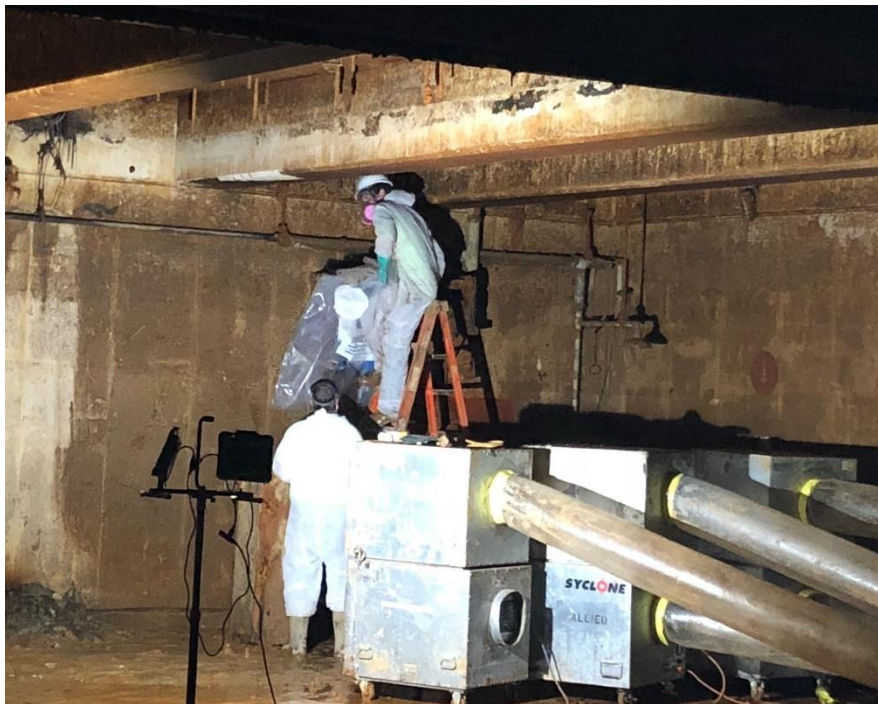
Photograph 12: Asbestos removal inside Silo 5 (7/10/18).
