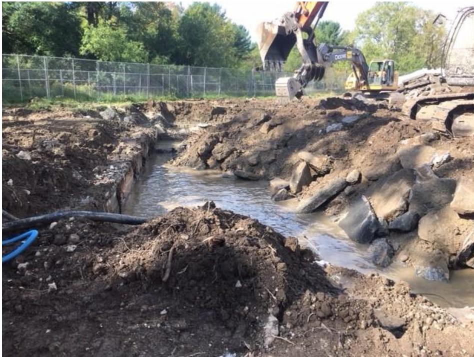
Photograph 22: Excavation and dewatering at previously demolished Silo 6 (9/20/18).
