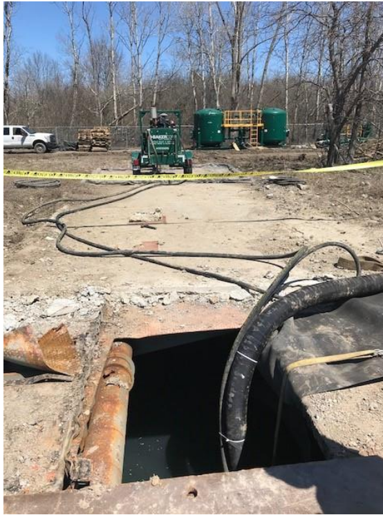
Photograph 3: Dewatering Silo 2 (4/23/18).
