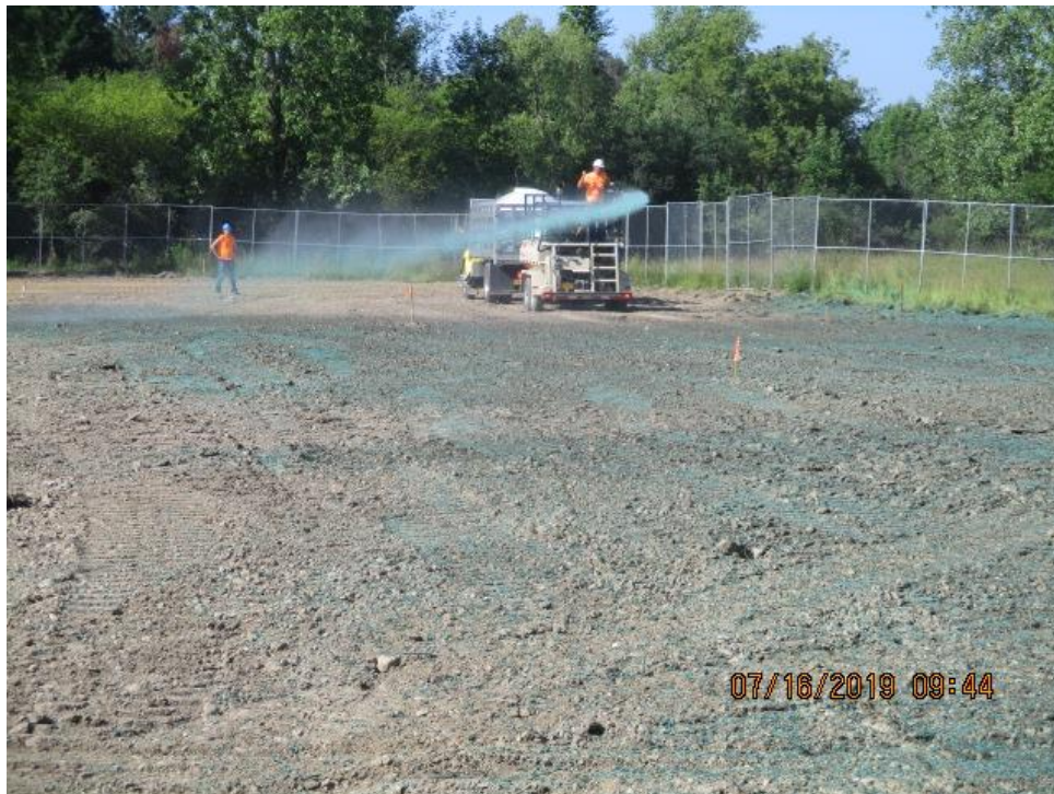
Photograph 54: Hydroseeding site (07/16/19).
