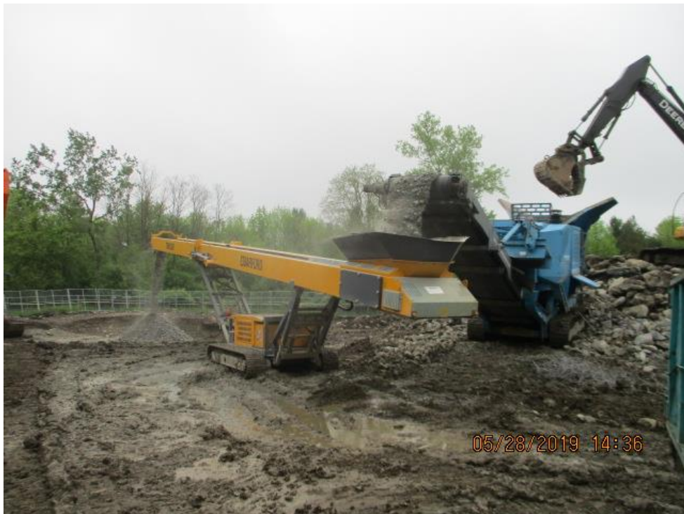
Photograph 42: Crushing concrete into smaller sized pieces for use as backfill (05/28/19).
