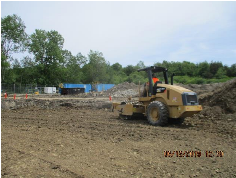
Photograph 46: Backfill Silo 2 with imported fill (06/12/19).
