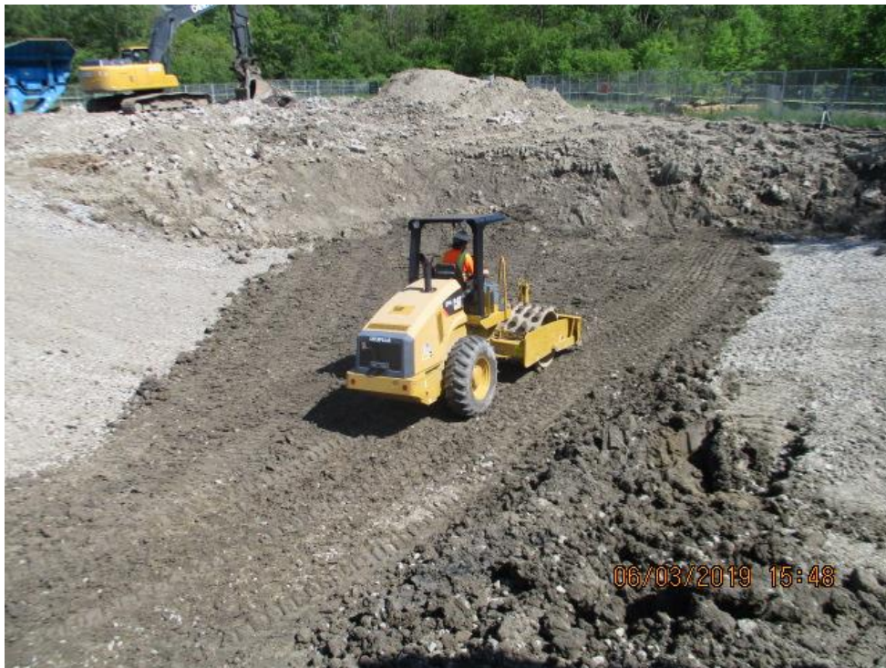
Photograph 44: Backfill Silo 5 with native soil (06/03/19).
