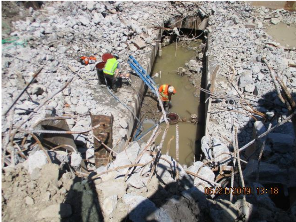
Photograph 41: Pumping hydraulic oil from elevator piston assembly (05/21/19).
