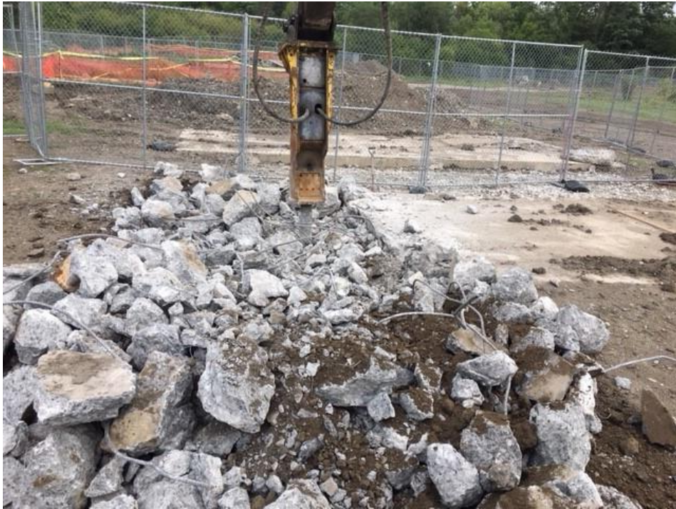
Photograph 19: Hammering concrete launch pad at Silo 2 (8/22/18).
