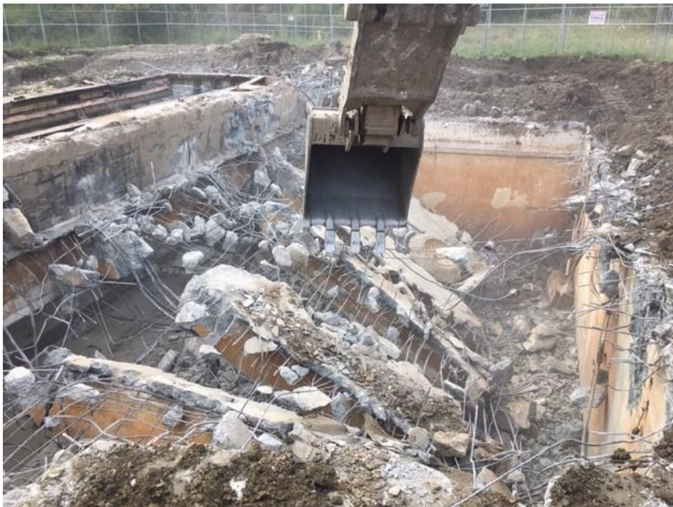
Photograph 24: Demolition of support beams and elevator door platform at Silo 4 (10/10/18).
