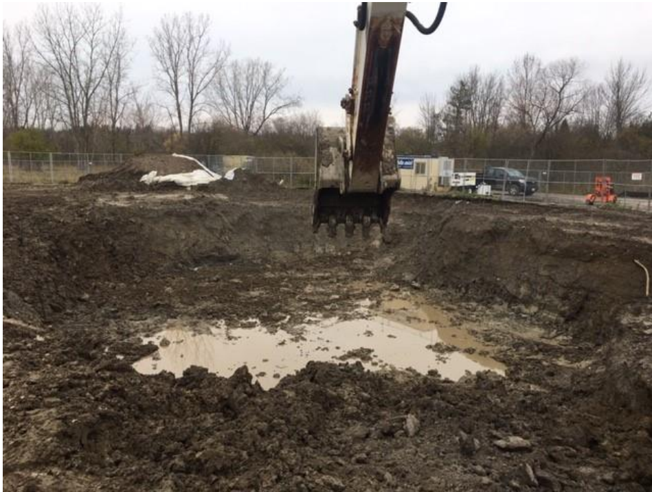
Photograph 29: Backfill with soil and crushed concrete at Silo 1 (11/12/18).
