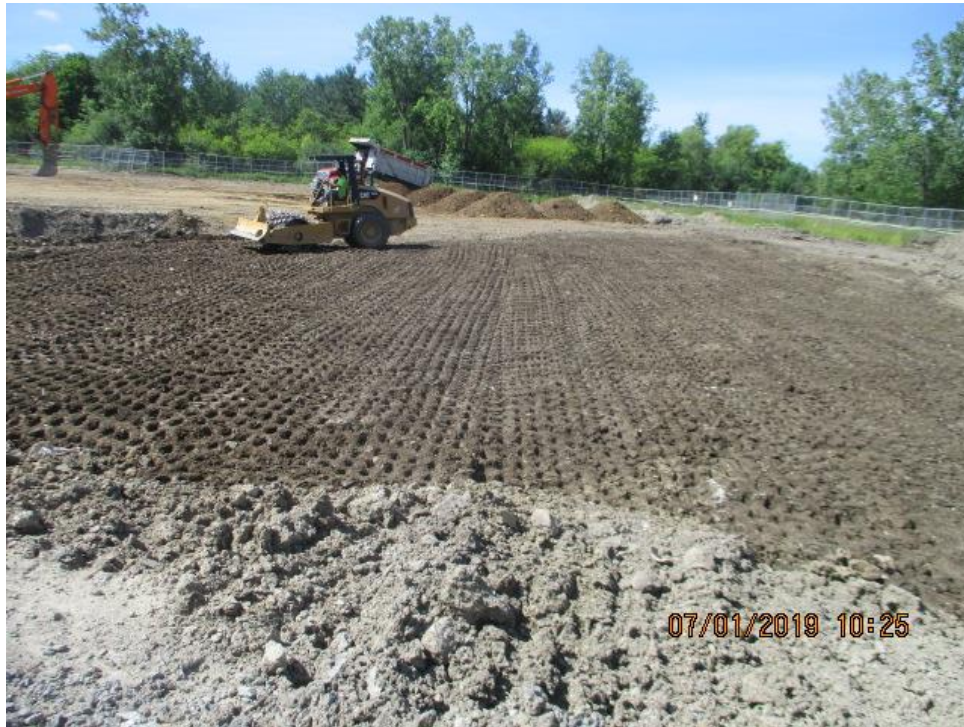
Photograph 49: Backfill compaction of former silo area (07/01/19).
