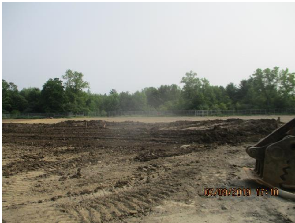
Photograph 52: Placement of native topsoil (07/09/19).
