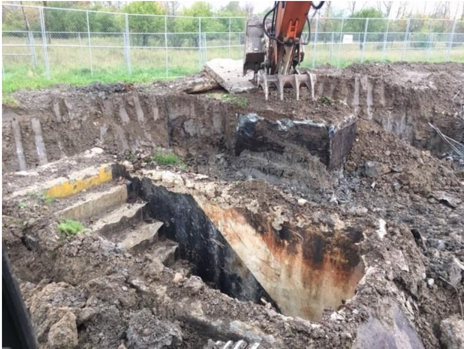
Photograph 25: Excavation around personnel room and stairwell at Silo 4 (10/11/18).
