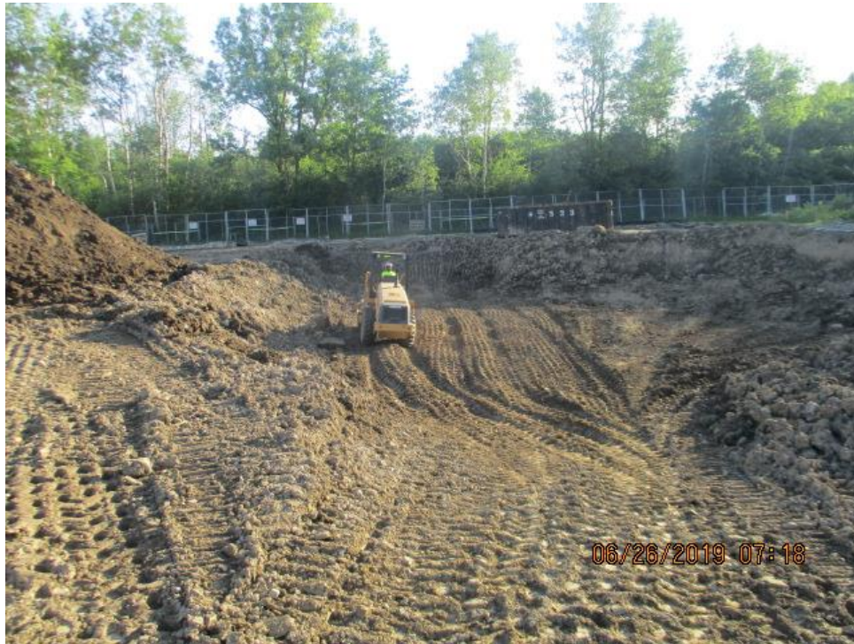
Photograph 47: Compaction of silo (06/26/19).
