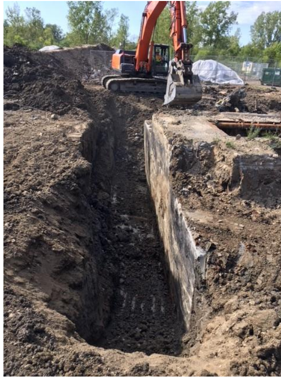
Photograph 21: Excavation of side wall at Silo 2 and covered soil pile (9/4/18).
