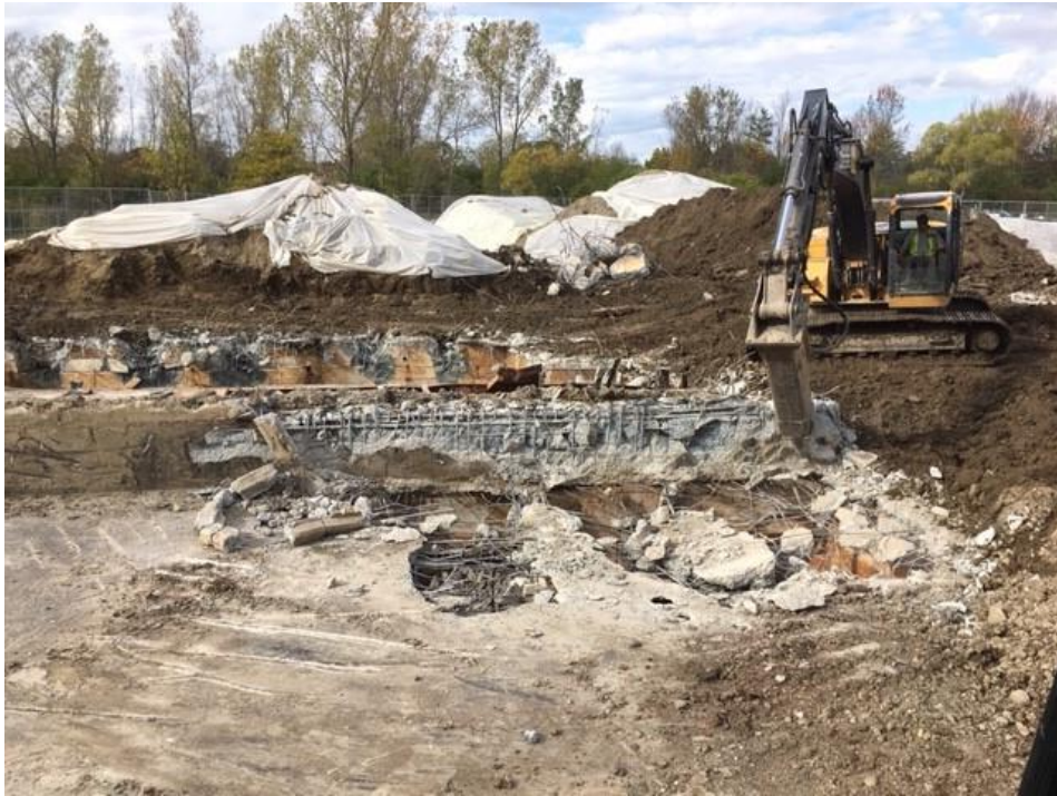
Photograph 23: Demolition of side walls at Silo 4 (10/10/18).
