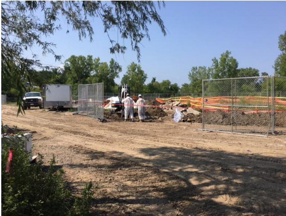
Photograph 17: Excavation to remove asbestos containing transite piping from Silo 1 (8/6/18).
