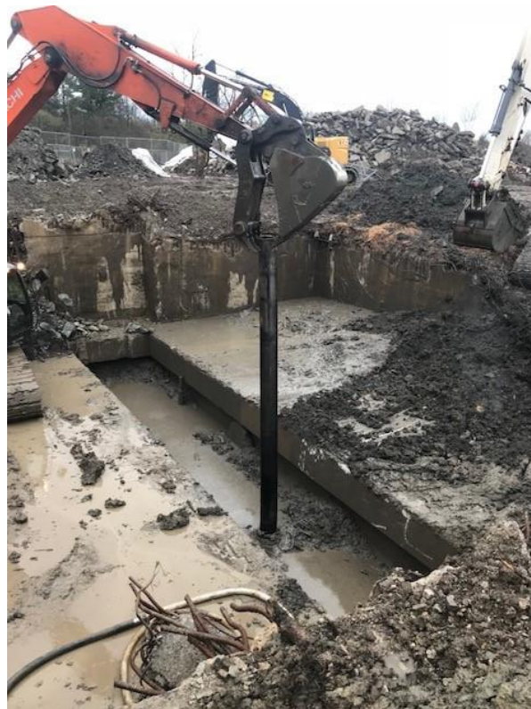
Photograph 26: Removing elevator piston at Silo 6 (11/6/18).
