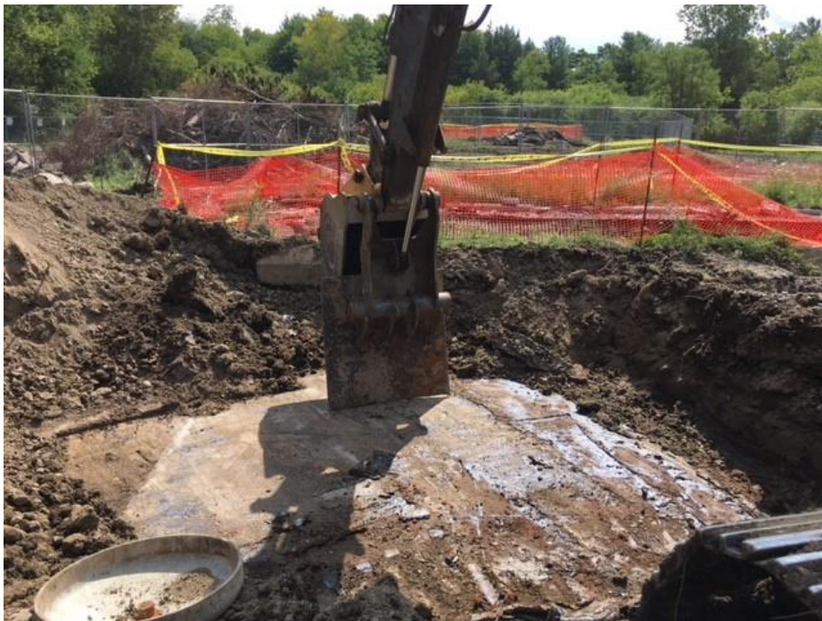
Photograph 18: Roof coating removal from Silo 2 (8/9/18).
