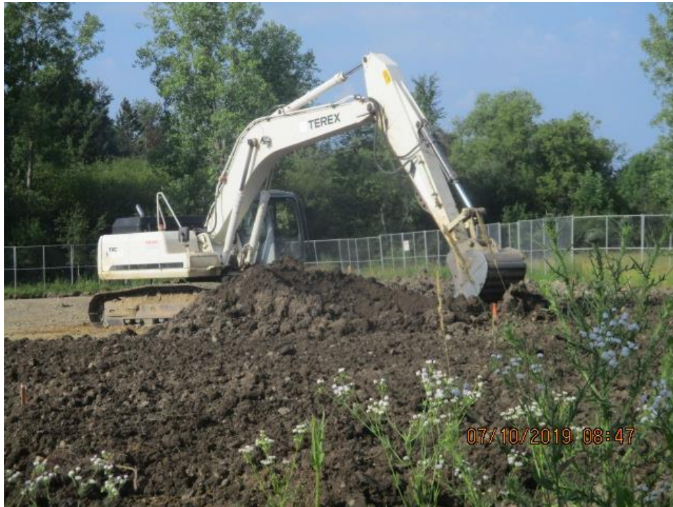
Photograph 53: Native topsoil placement (07/10/19).
