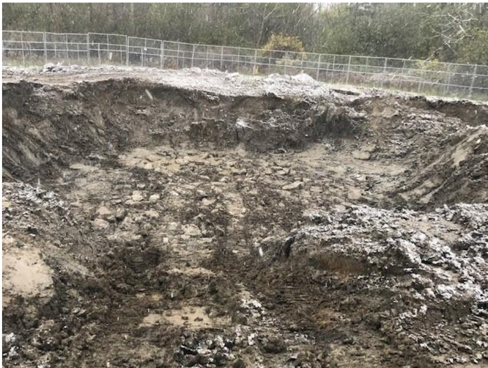
Photograph 30: Backfill with soil and crushed concrete at Silo 6 (11/13/18).
