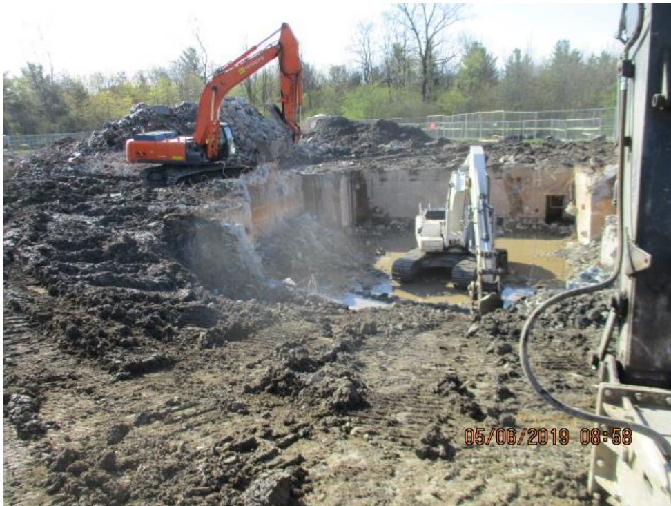
Photograph 38: Demolition of walls at Silo 5 (05/06/19).
