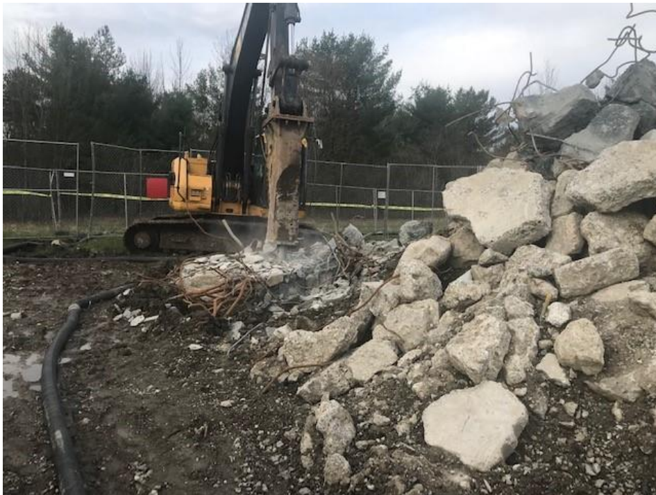
Photograph 34: Concrete crushing to reduce concrete size (04/23/19).
